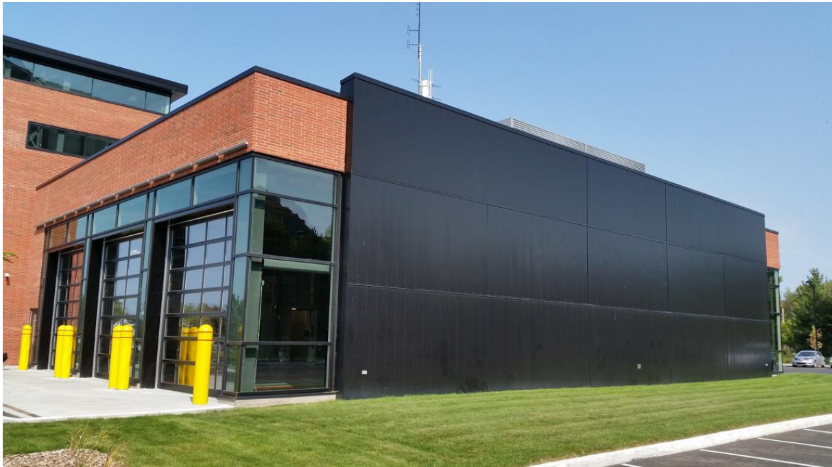
New-built firehall south of Montreal with a south-facing solar air heating wall for preheating the incoming fresh air during the heating season. Photo: Matrix Energy
