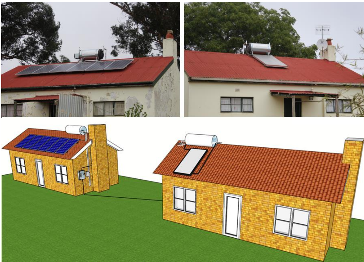
Figure 1: PV hot water and SWH system installed at Mariendahl Farm residence in Western Cape, South Africa (SketchUp Free)
