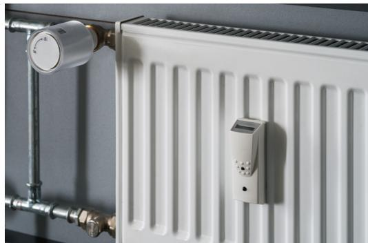
The thermostatic valve is the last control unit of a DDS; the customer sets the desired temperature for each room of their apartment with thermostatic valves. Only with thermostatic valves can the full potential of efficiency measures be realised. **The whole package of technical equipment including heat substations, thermostatic valves and HCAs, is a functional unit.**
