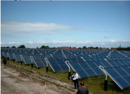
43 44 Figure 1. Solar collector field with a high number of rows with flat plate collectors.
