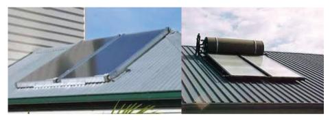
Figure 6.2: Flat Plate collector mounted on ordinary galvanized and box-type iron sheet roofs (Refer to Figure 5.9 for installation guideline)
