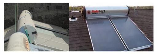
Figure 6.4: Storage tanks and collectors mounted on rooftops
