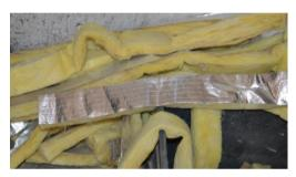
*Figure 4.14: Fibre glass linings with aluminium foiling – by steelstone*
