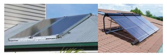
Figure 6.3: Collector and evacuated tube mounted on roof tops
