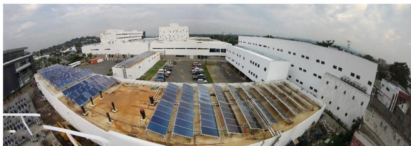
**Fig. 4: Panorama view of 4450 m<sup>2</sup> collector area installed at Managua Hospital, Nicaragua.**
