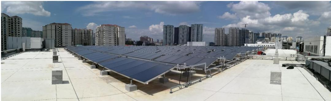
Fig. 6: Panorama view of 2472m<sup>2</sup> collector area installed at IKEA.
