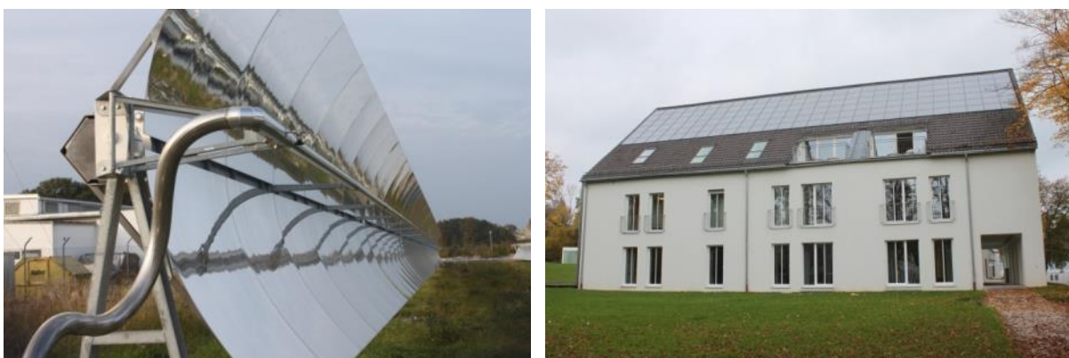
Figure 9: Parabolic trough solar thermal research plant (left) as well as a roof-top solar collectors connected to a small district heating system in Bad Aibling, Germany (Source: Rutz D.)
