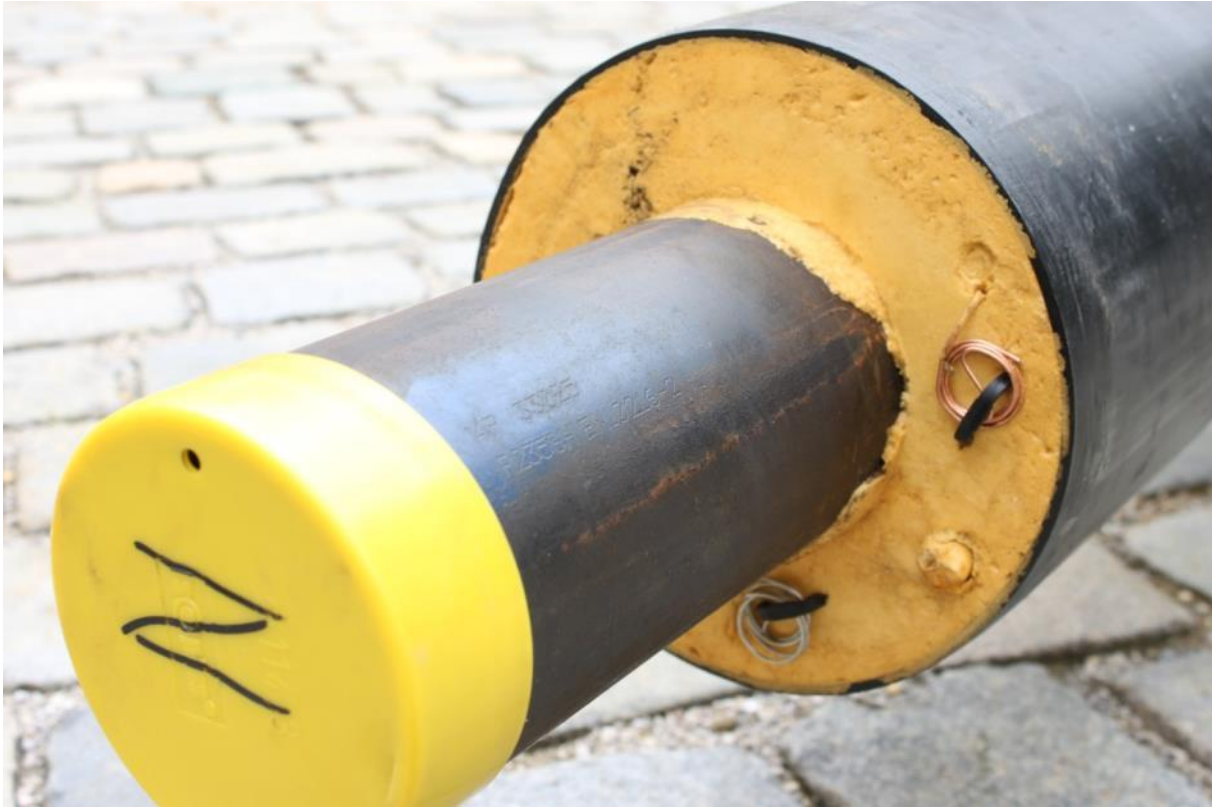
Figure 51: Single steel pipe with two wires for the leakage warning system (Source: Rutz D.)
