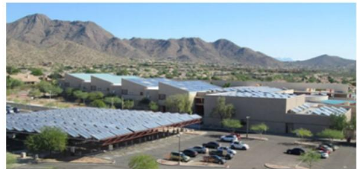
Solar heating and cooling
