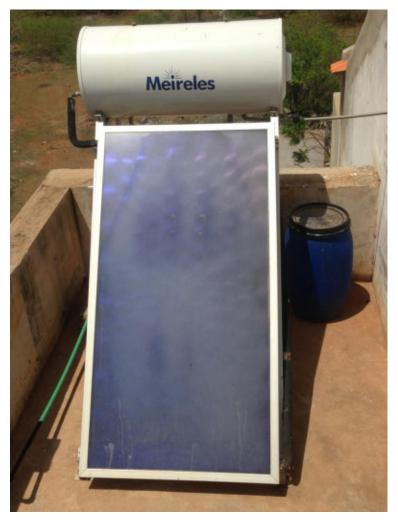
Figure 17: Thermosyphon system found on single family house of 4 persons with storage of 190 liters. On the 13 of September, 2015 at 13:50 local time a temperature of  $69.2\,^{\circ}\text{C}$  was recorded from the outlet of storage tank. Positioning of the collector is not optimized (>45 degrees) because of lack of space.
