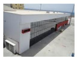
Figure 24: Passenger Maritime Station of Porto Novo, Santo Antão – south and west façade glassed. The installed AC units revealed inadequate during operation. AC Condensers placed in the searing heat of the roof.
