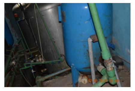
Figure 10: MINDEL Hotel – storage tanks and distribution piping uninsulated
