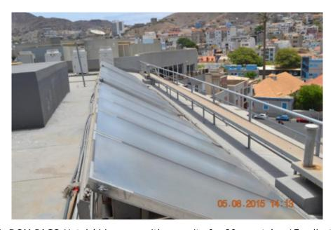
Figure 7: DOM PACO Hotel (44 rooms with capacity for 80 guests) – 15 collectors from CPC AO SOL with individual area of 2.51 m2, or 37.65 m2 equivalent to 26.4 kW. The system supplies hot water to rooms, laundry and kitchen services.
