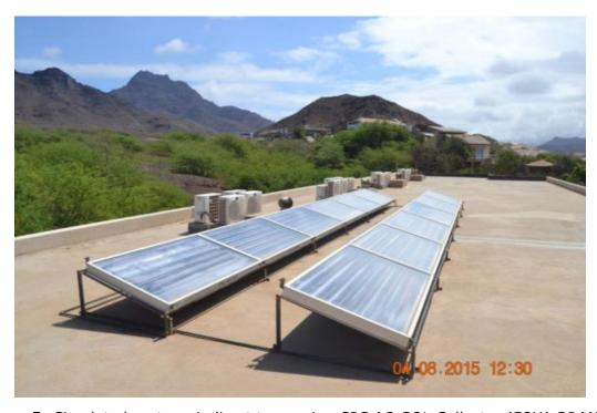
Figure 5: Circulated system, indirect type using CPC AO SOL Collector (FOYA BRANCA Hotel, in S. Vicente
