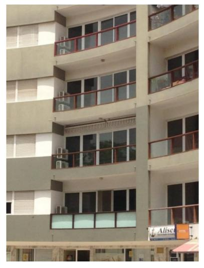
Figure 27: Condensers of compression type AC units in real estate investment in S. Vicente
