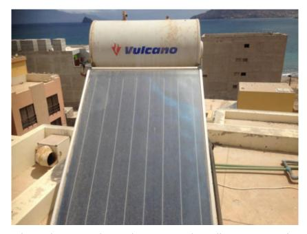
Figure 3: 150 liters thermo syphon indirect type solar collector mounted in small hotel Alternatively, some small hotels use direct type solar water heater of 135 liters.
