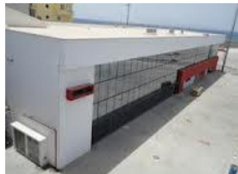
Figure 24: Passenger Maritime Station of Porto Novo, Santo Antão – south and west façade glassed. The installed AC units revealed inadequate during operation. AC Condensers placed in the searing heat of the roof.
