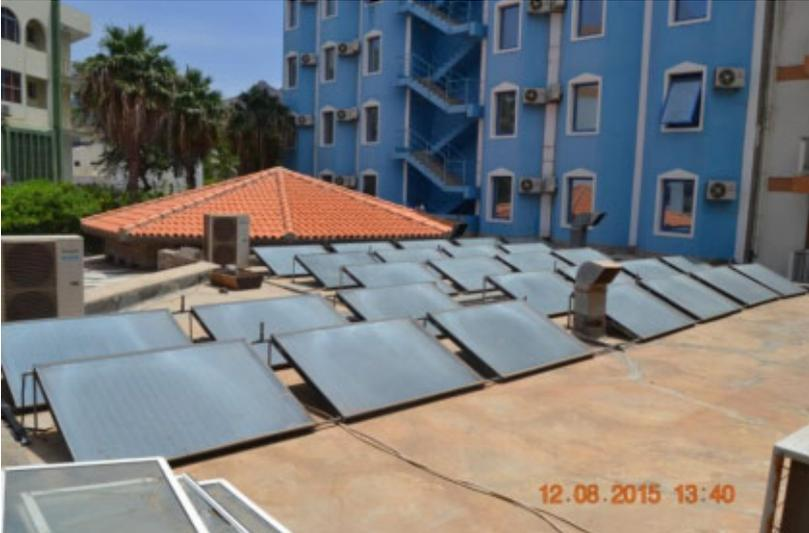
Figure 8: MINDEL Hotel flat plate solar collector (1.7 x 1.2 m) unbranded Italian made
