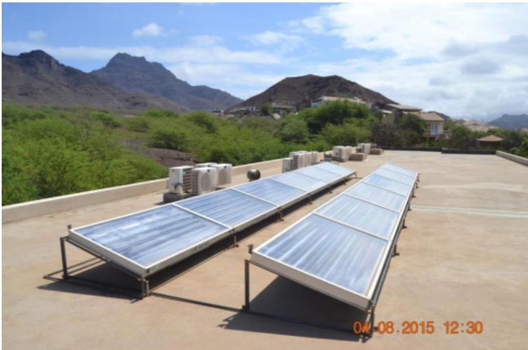
Figure 5: Circulated system, indirect type using CPC AO SOL Collector (FOYA BRANCA Hotel, in S. Vicente)
