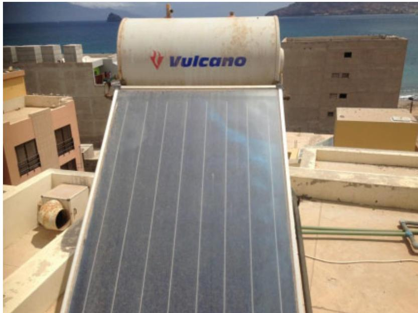
Figure 3: 150 liters thermo syphon indirect type solar collector mounted in small hotel
