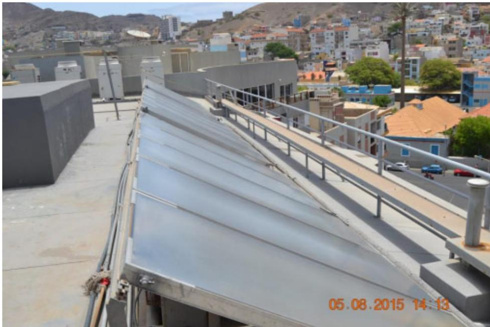
Figure 28: CPC AO SOL collector field mounted in a metal structure on the terrace of Dom Paco Hotel
