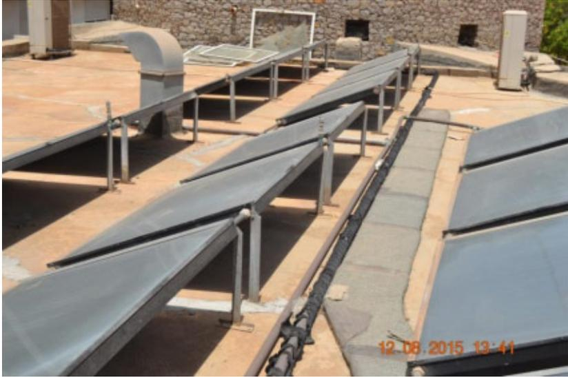
Figure 9: MINDEL Hotel, poorly insulated copper piping carrying hot water to storage tank
