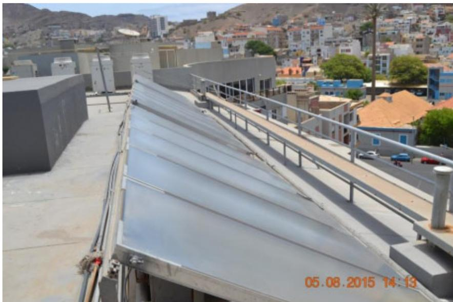
Figure 7: DOM PACO Hotel (44 rooms with capacity for 80 guests) – 15 collectors from CPC AO SOL with individual area of 2.51 m<sup>2</sup>, or 37.65 m<sup>2</sup> equivalent to 26.4 kW. The system supplies hot water to rooms, laundry and kitchen services.
