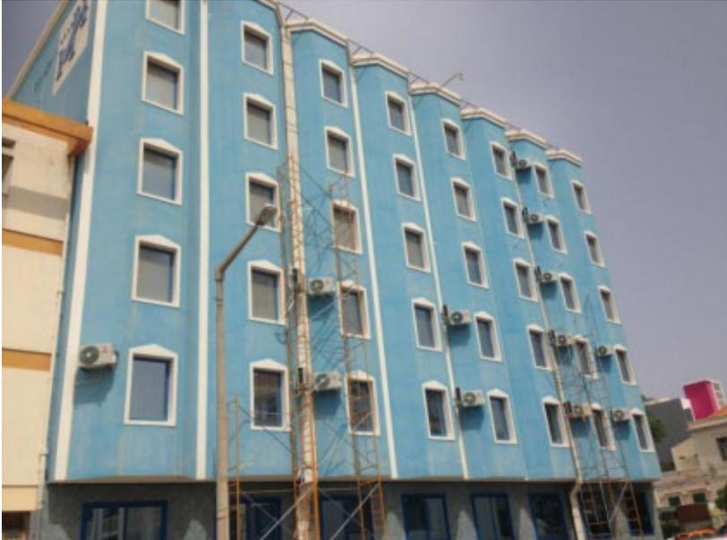
Figure 26: Condensers of compression type AC units being mounted in a hotel in S. Vicente (damaging the façade aesthetic)
