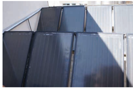
Figure 3 Collectors partly shadowed in the afternoon
