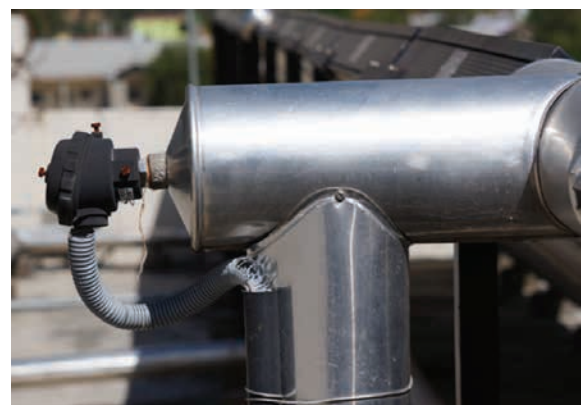
Figure 6 Collector outlet temperature sensor is located in the pipe close to the collector outlet.
