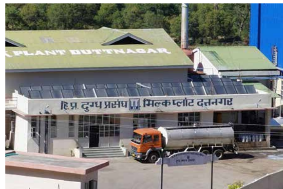
Figure 2 Orientation of the collectors towards south-east due to installation area
