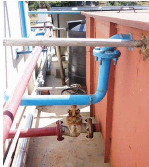
Figure 4 Boiler feeding water tank (right side) with pipe from the solar system (blue) and the pipe to the boiler (red)
