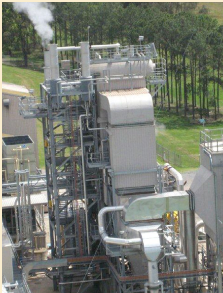
Installation of the new 45m stack and the Fluidised bed boiler at the Nescafé factory, photos CPM Engineering and Nestlé Australia
