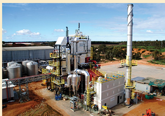
Automatic feed handling and 8MW th boiler using grape marc, photos Australian Tartaric Products
