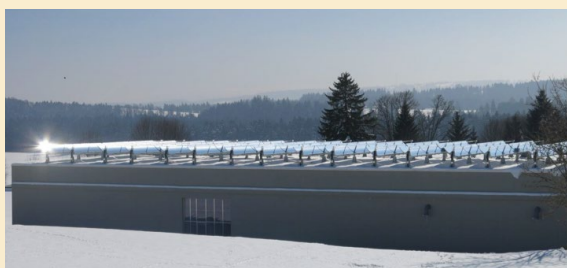
Parabolic trough collector in Switzerland and a ground-mounted system in Newcastle, photos NEP Solar
