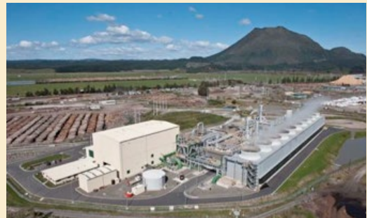
Kawerau timber mill site and 8.3MW binary cycle plant installed in 2008, photos NZ Geothermal Association
