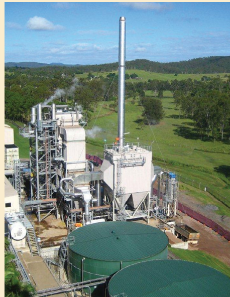
Installation of the new 45m stack and the Fluidised bed boiler at the Nescafé factory, photos CPM Engineering and Nestlé Australia
