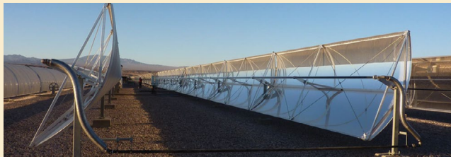
Parabolic trough collectors and thermal storage tanks at Minera El Tesoro, photos Abengoa Solar
