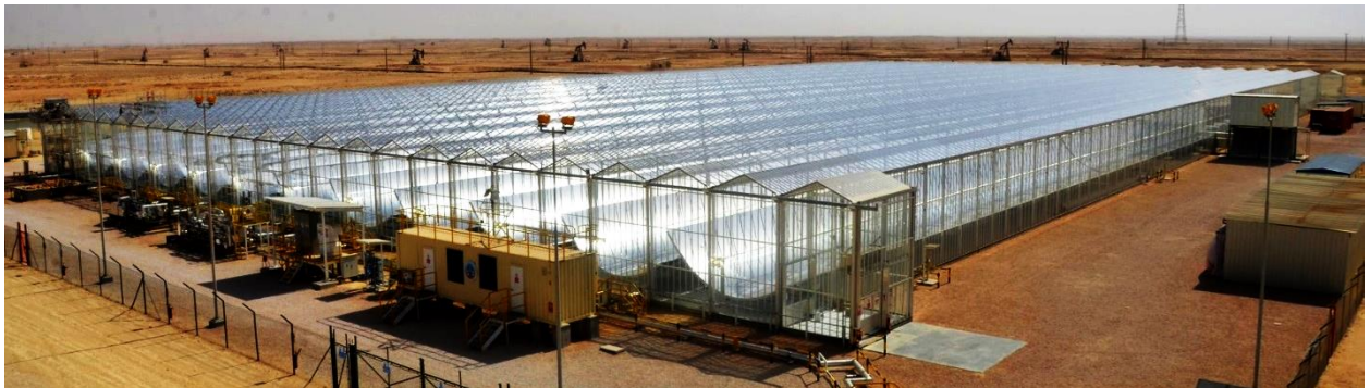
Figure 2: GlassPoint pilot plant, South Oman
