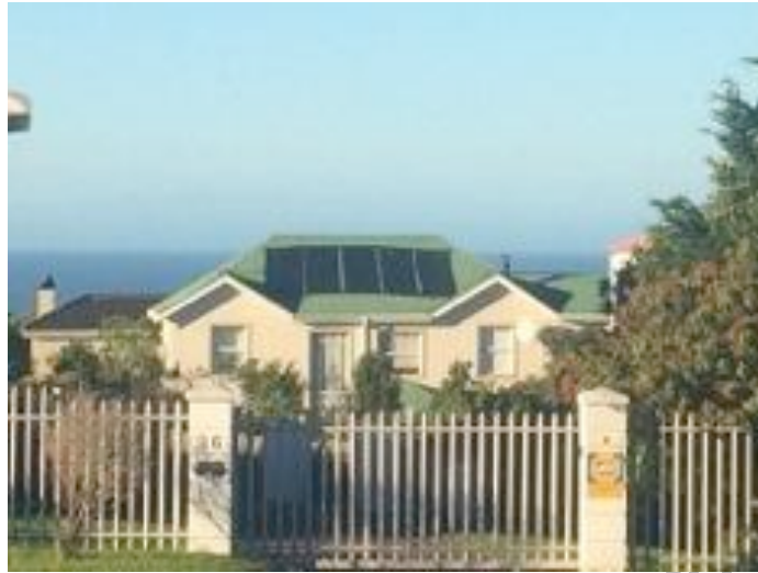
Figure 11: Typical rooftop installation of an unglazed swimming pool heater in South Africa
