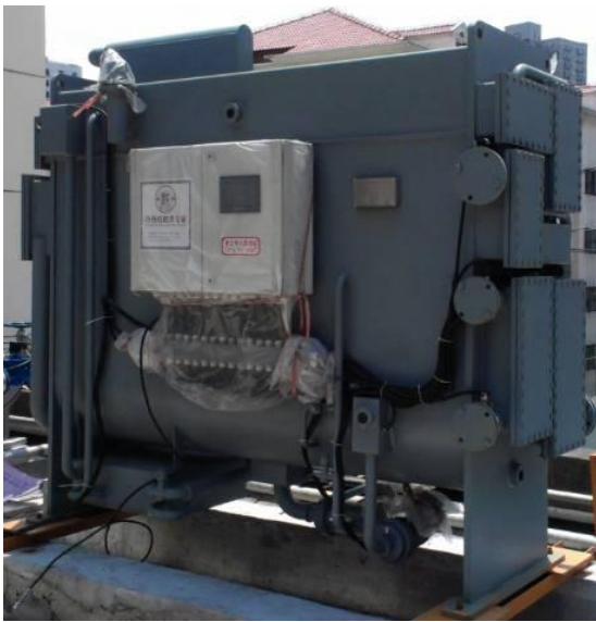
Fig.7 Single/Double effect absorption chiller for solar cooling
