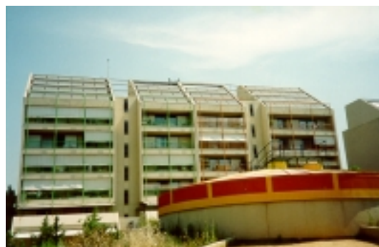
Lykovrissi: the interseasonal storage tank in front of the heated building.
