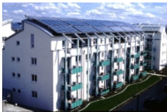
2 700 m 2 (+ 1 550 m 2 extension in progress) collector array in Friedrichshafen 1996. Photo: Boris Mahler.
