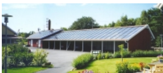
220 m 2 roof module collectors in Onsala. Photo: Jochen Dahm
