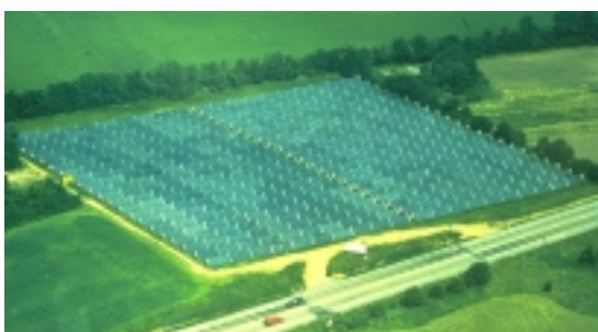
5 500 m 2 collector array in Falkenberg 1989. Photo: Falkenberg Energi AB.
