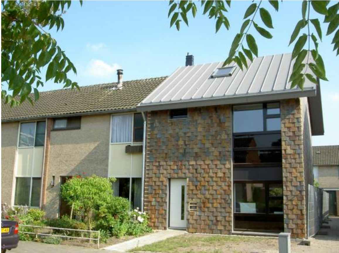
Figure 7: A test house has been built before the large scale renovation took place to get used to the renovation method and details
