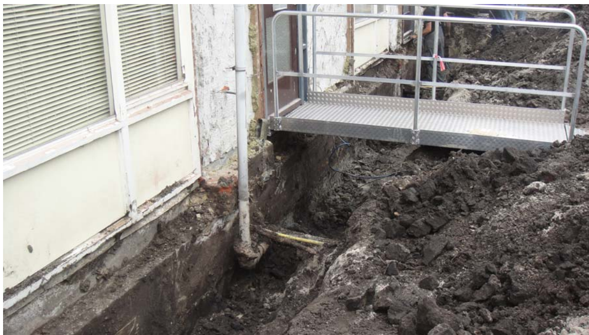
Figure 10: Ditch around the houses to prepare for foundation works and perimeter insulation
