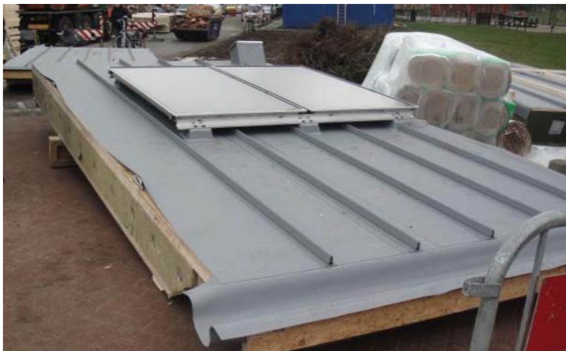
Figure 14: The solar collector and roofing material were pre-installed in the factory
