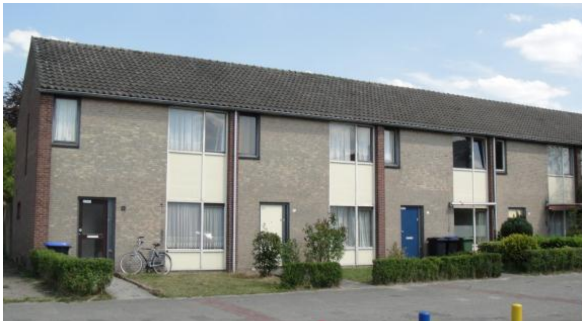
Figure 3: Front elevation before renovation
