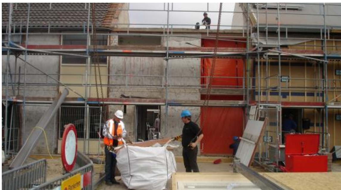
Figure 15: The one day in which the roof and windows were dismantled (middle house). At the end of this day the house was weather and watertight with mounted roof and façade elements
