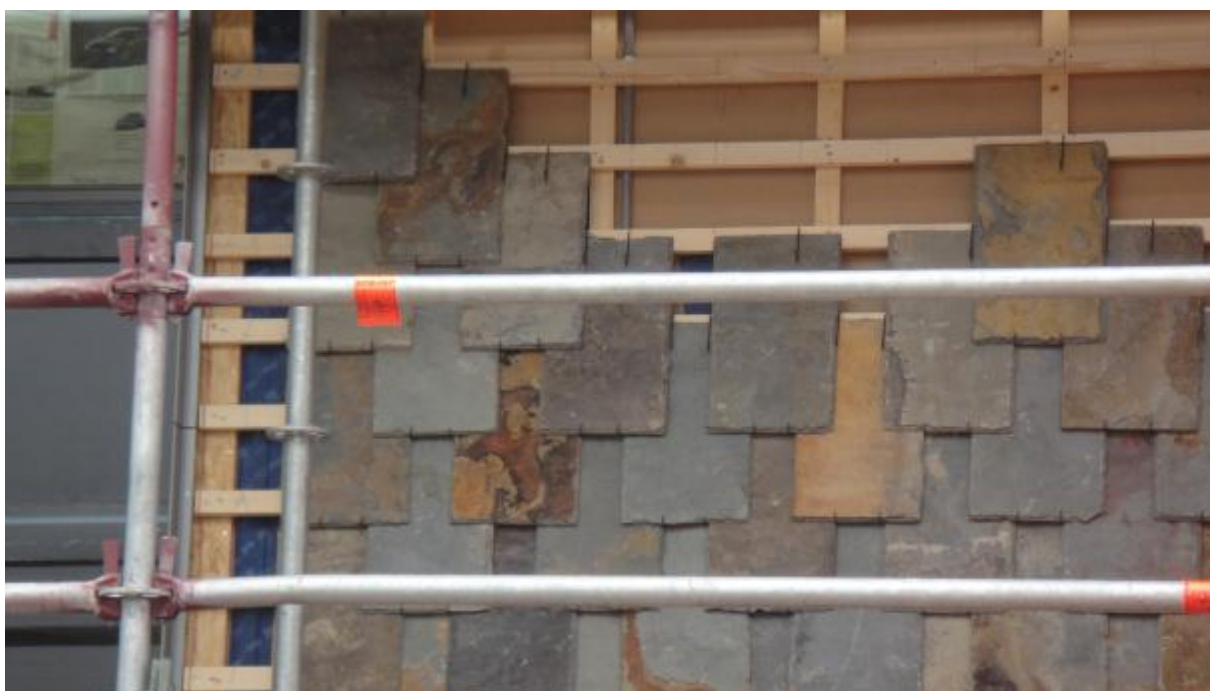
Figure 22: Detail of façade cladding with natural slates, which was chosen by the architect
