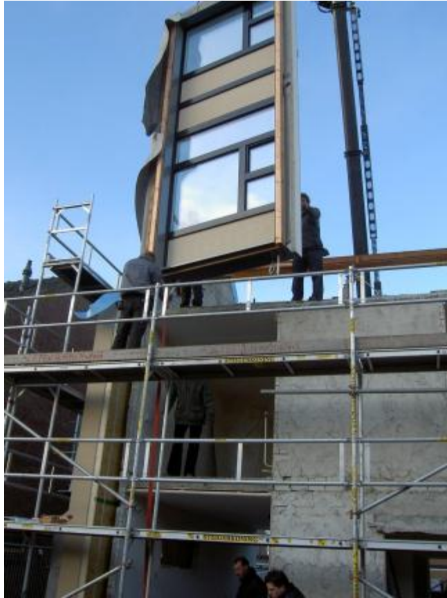
Figure 8: Mounting of prefabricated façade element
