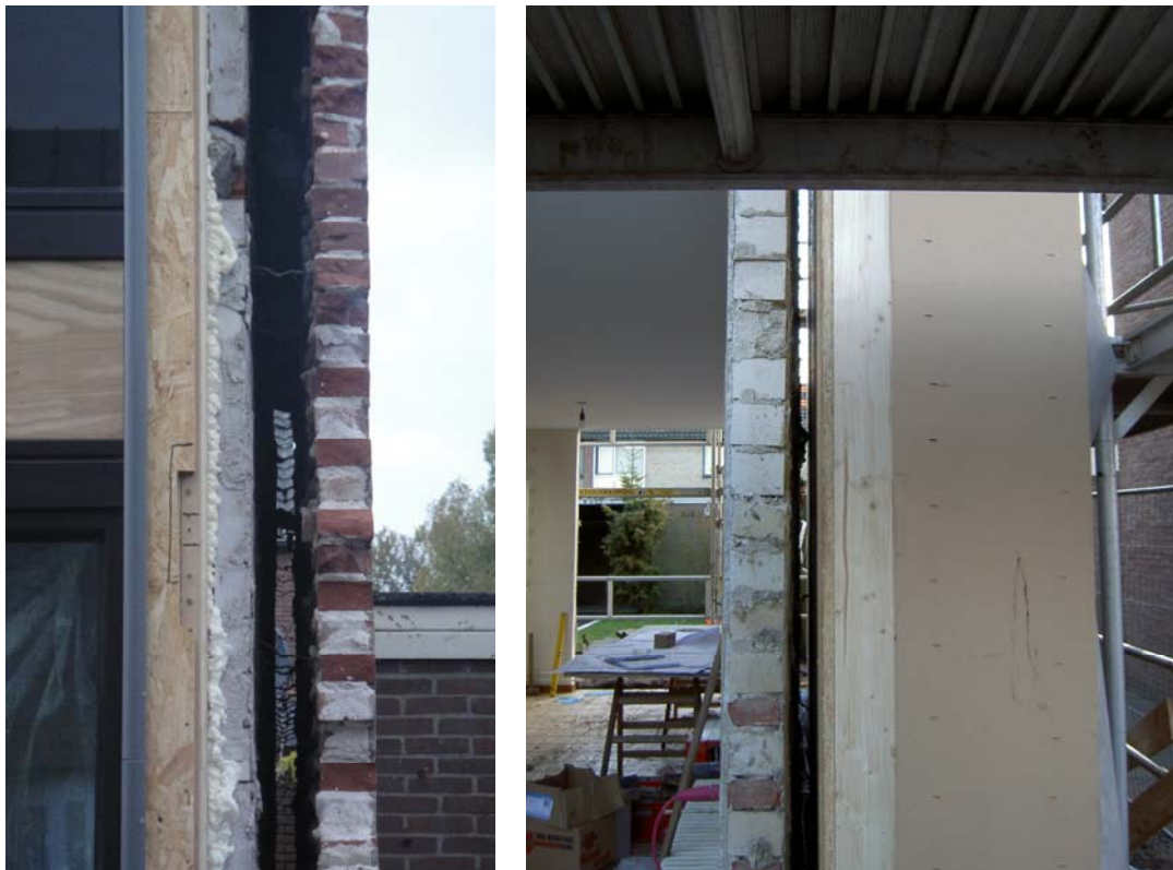
Figure 9: Left: cross section of existing cavity wall. Right: cross section after placement of prefabricated façade element.
