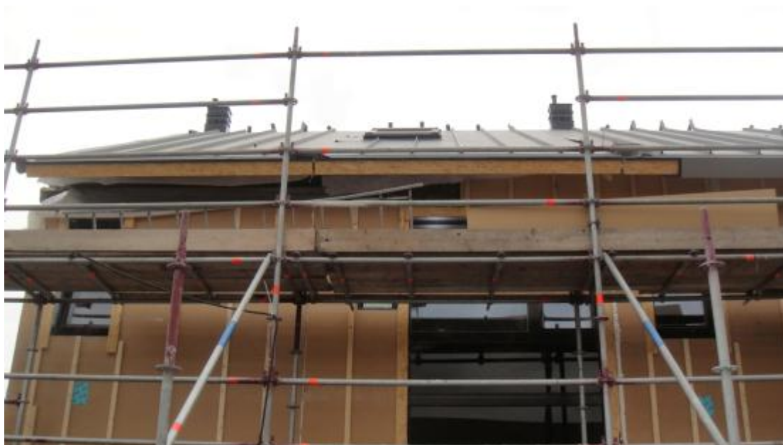
Figure 17: The gap between façade and roof element was filled in situ
