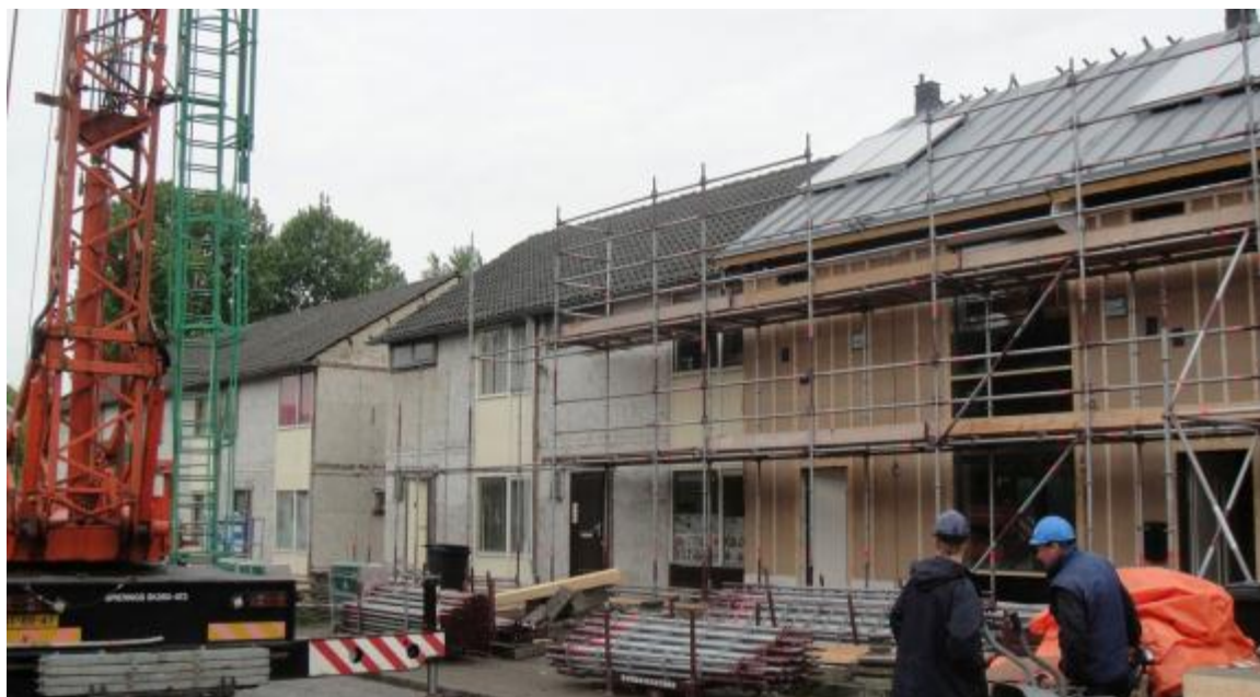
Figure 16: The renovation process continued as a train through the area: 4 houses in a week
