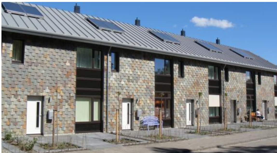
Figure 5: Front elevation after renovation
