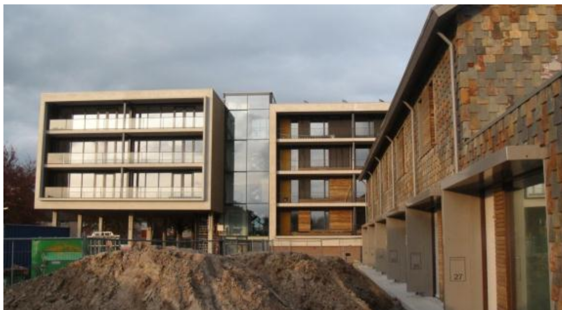
Figure 24: In the period 2011 – 2013 new construction took place in the same area, which was also passive houses, designed in the same style as the renovation houses.
