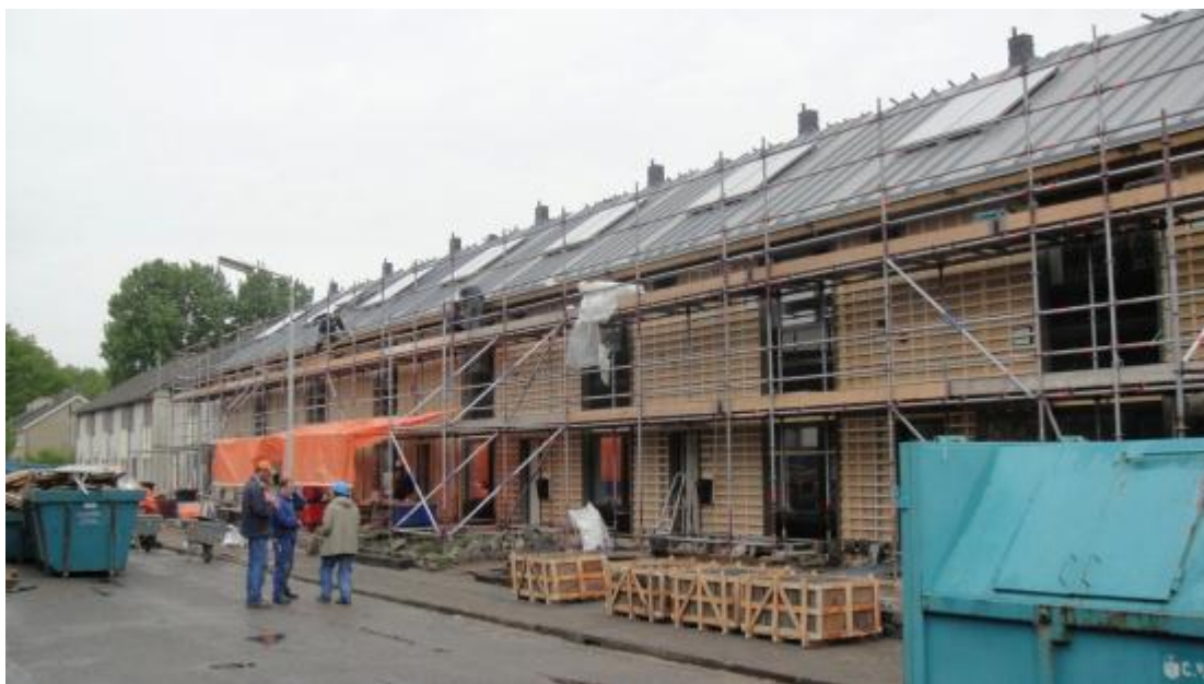
Figure 21: External façade cladding works for a completed block of houses
