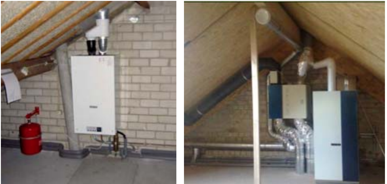
Figure 19: Left: condensing gas boiler before renovation; Right: the new compact system includes a mechanical heat recovery unit, a condensing gas boiler, and a storage tank – connected to the solar collectors.
