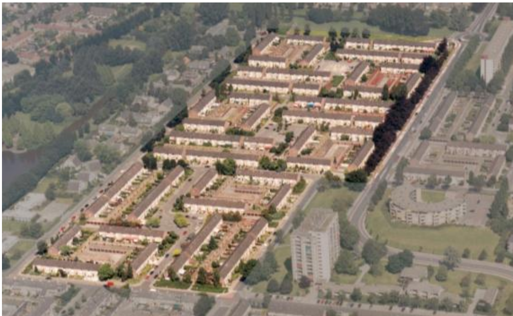
Figure 1: Part of the district Groot Kroeven, Roosendaal before renovation
