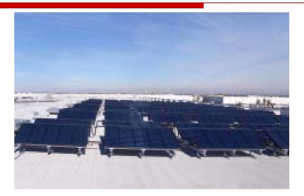
Solar Water heating for Industrial processes. One the biggest solar process heat system in North America - 893 m<sup>2</sup>/9600 ft<sup>2</sup>
