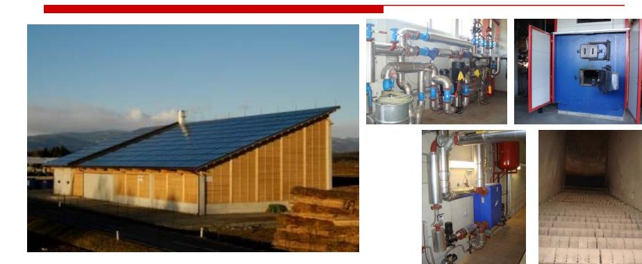
District heating system + using heat to dry wood chips. Solar water heating covers most of the summer load on the district heating grid. Solar panels 1300 m<sup>2</sup>/13875 ft<sup>2</sup>, 90m<sup>3</sup> buffer tank
