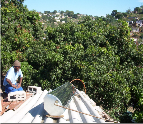
Figure 6: Typical integral SWH installations
