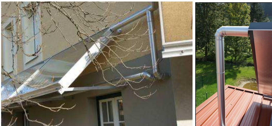
Figure 79: External pipe insulation (Source: AEE INTEC / Austria): good quality of insulation and protection
