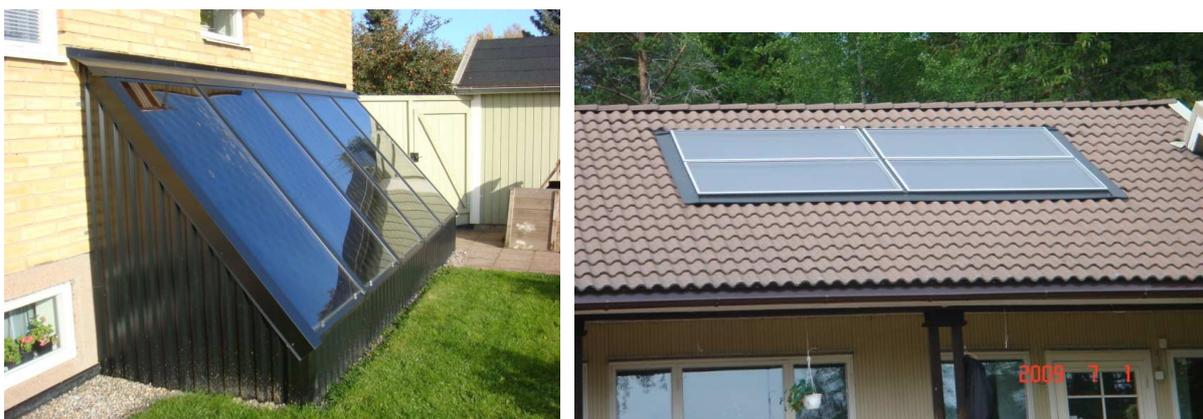
Figure 30: Examples of collector mounting (Source: SERC / Sweden)
