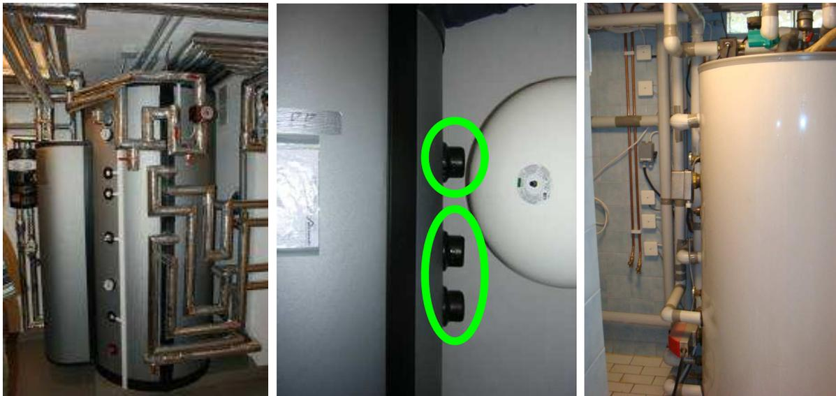
Figure 46: Heat storage with thermosiphon heat traps at all pipe connections and all pipes insulated (left), prefabricated insulation elements for unused pipe connections (middle), pipes connected at the tank are good insulated completely to the tank (right).
