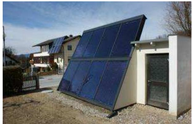
Figure 31: Examples of collector mounting (Source: AEE INTEC / Austria)
