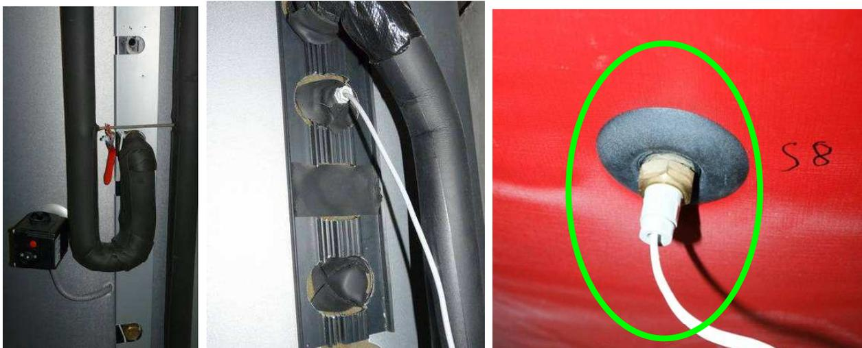
Figure 76: Example of good/acceptable installation details: insulated thermosiphon heat trap (left, Source: INES Education); basic insulation of temperature sensor and unused pipe connections (middle, Source: INES Education); temperature sensor well fixed and pipe for immersion sleeve insulated (right, Source : AEE INTEC)
