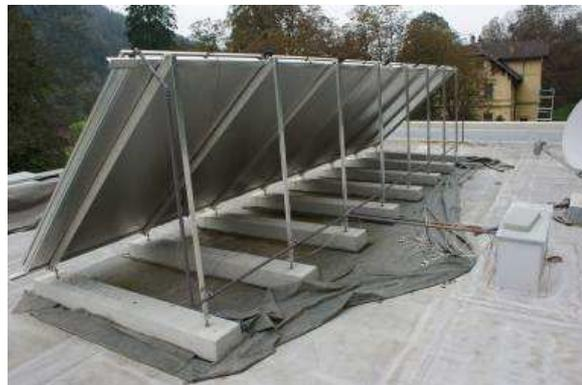
Figure 36: External pipe insulation (Source: AEE INTEC / Austria): left side: partly no insulation and no protection; right side: absolutely no insulation, therefore nothing which could be protected ☹
