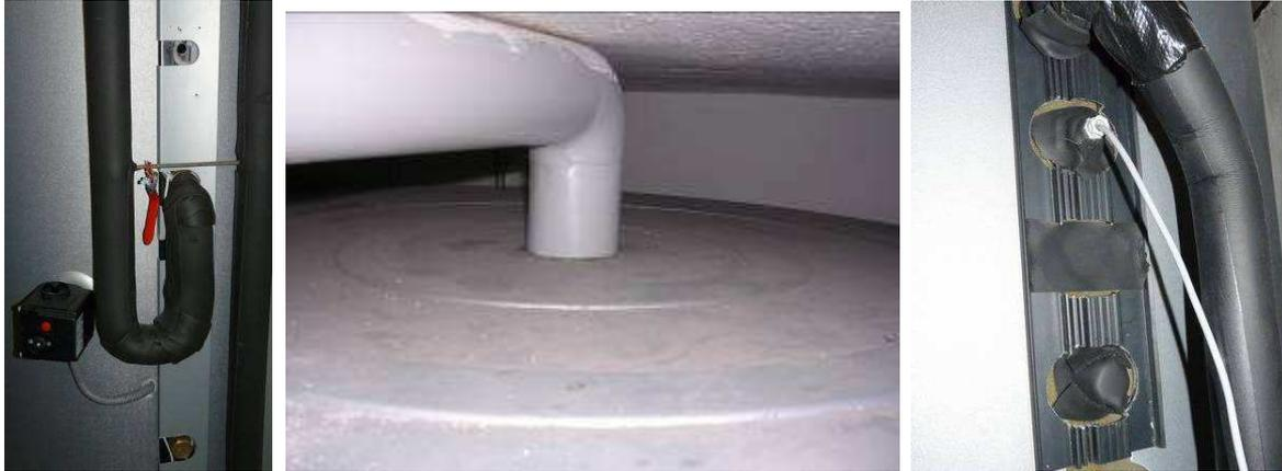
Figure 45: Perfect insulated thermosiphon heat trap (left), good closed top tank insulation and insulated pipe connection (middle), pipe connection downwards and insulated temperature sensor immersion sleeve and insulated unused pipe connections (right).
