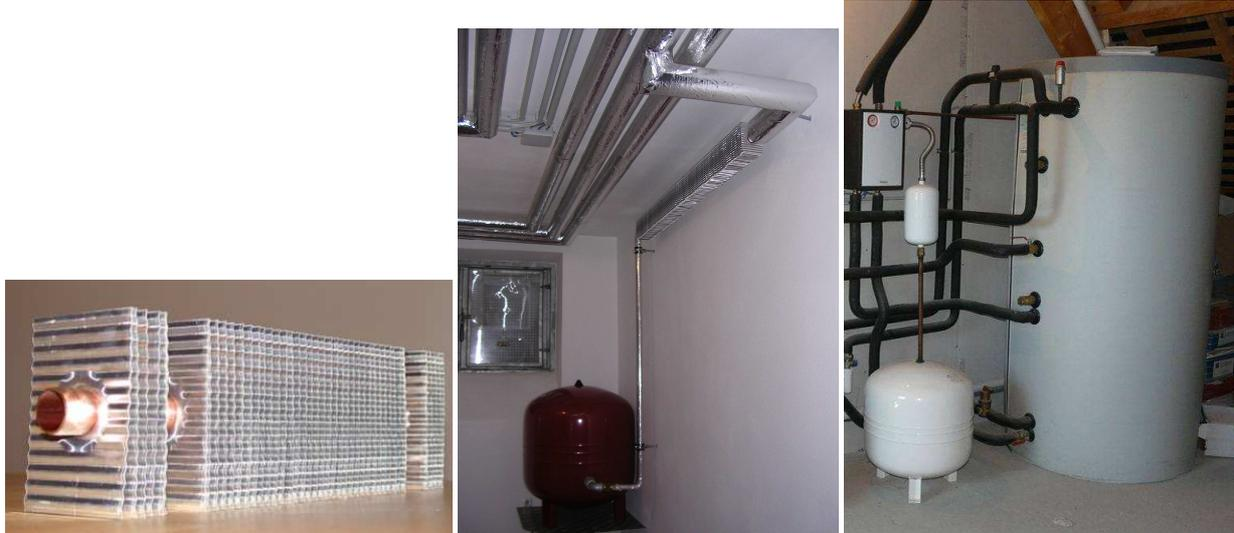
Figure 81: Stagnation cooler, performed as a baseboard heating fitting (left) and mounted (middle) or “preposition vessel” (right)
