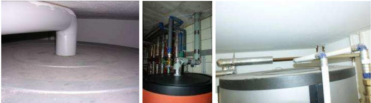
Figure 75: Examples of good insulated top of heat storages and best case (right) of a totally closed top insulation of a heat storage.
