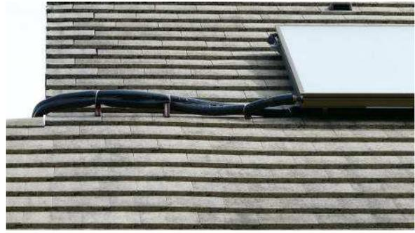
Figure 34: External pipe insulation (Source: Ines Education / France): left side good quality of insulation and protection; right side well insulated but no protection.
