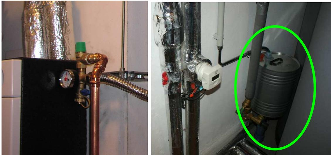
Figure 85: Drain pipe at outlet of pressure relief valve made of copper (left) and collection tank which is closed and made of metal (right)
