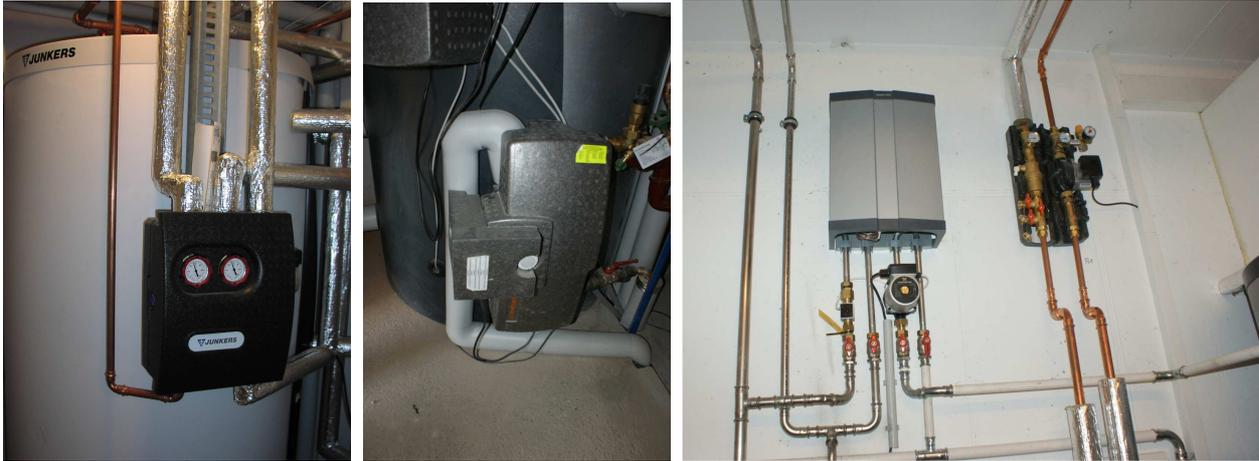
Figure 51: External Heat exchanger modules direct mounted at the tank (left and middle) or extra mounted at the wall (right).
