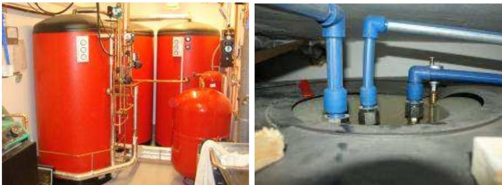
Figure 43: Multistore system in Sweden (left), bad top insulation of a tank in tank system in Austria (right).
