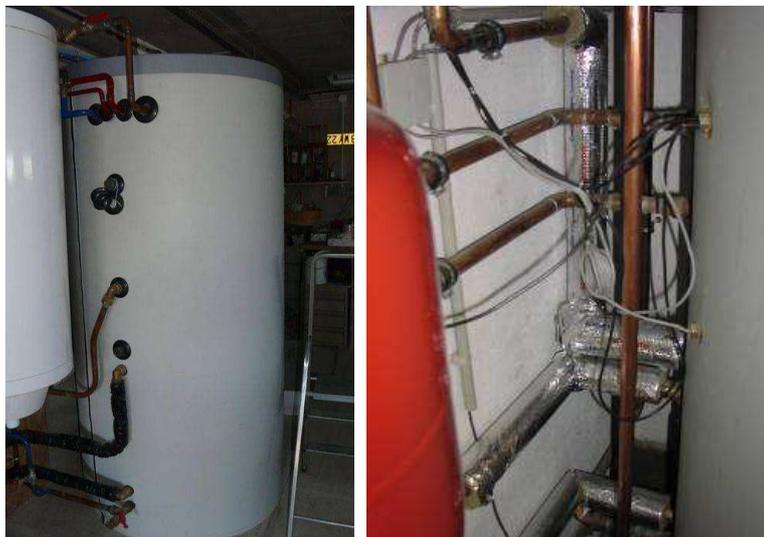
Figure 44: Not insulated and upwards connected pipes at the top of a tank in France (left), not insulated pipe connections and cold bridges due to temperature sensors at a tank in Germany (right).
