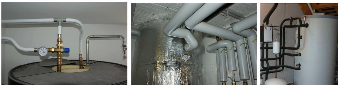
Figure 50: Heat storage insulation quality of tank in tank systems: pipe connections at top and bad (left) and good insulation (middle) or well insulated pipe connections at the side of the tank (right) which could be improved with pipes leading downwards immediately (thermosiphon heat trap).
