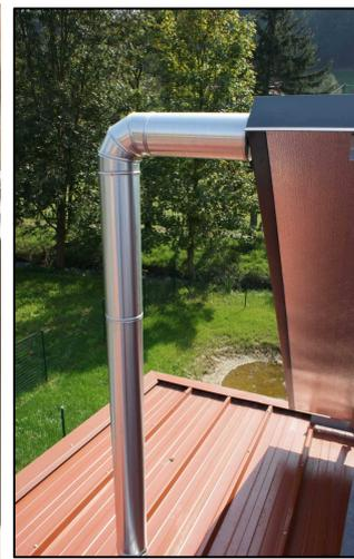
Figure 35: External pipe insulation (Source: AEE INTEC / Austria): good quality of insulation and protection
