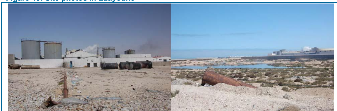
Figure 45: Site photos in Laâyoune
