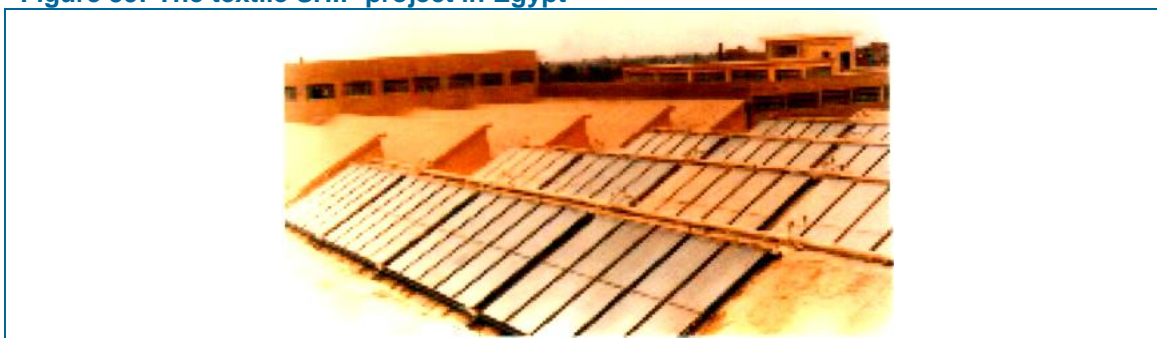
Figure 39: The textile SHIP project in Egypt
