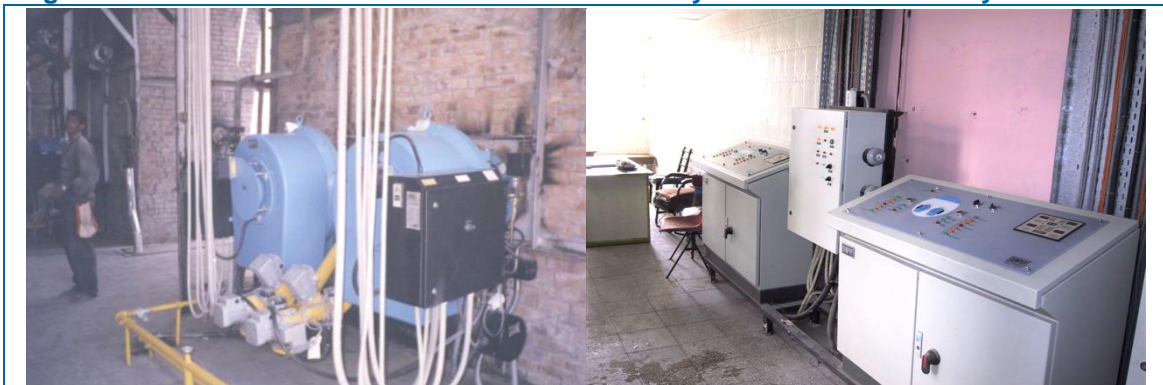
Figure 42: New dual burners with automatic control system in El Nasr factory
