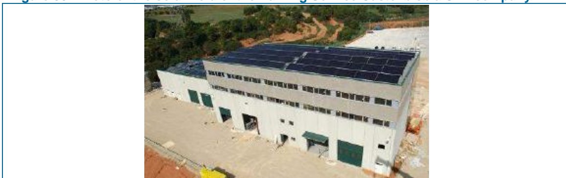
Figure 35: Photo of the solar field of the Parking Service Castellbisbla S.A. company
