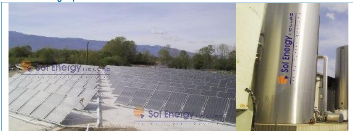
Figure 36: Photos of the Tyras S.A. thermal solar field installation (solar field -left- and tank boiler -right-)
