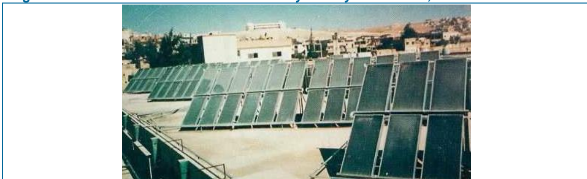
Figure 46: Solar thermal installation in a dairy factory in Russeifa, Jordan
