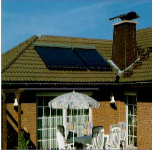
On sloping roof
