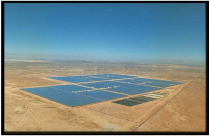
Solar central California (350 MW) 2
