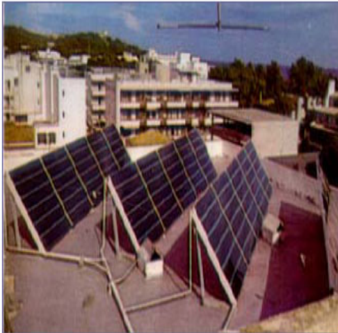
On flat roof
