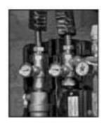
**Step 6:** If you are using single, 6' LineSets for connection to the tank from the pumping station, locate these now. If you are using copper piping from the pumping station to the tank, these connections to the solar storage tank can be made at this time.
