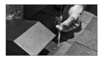
**Step 2:** For each collector, choose the intersections that match up with where your collectors will be mounted. The collector frame is designed to match up to rafters that are either 16" or 24" on center.
