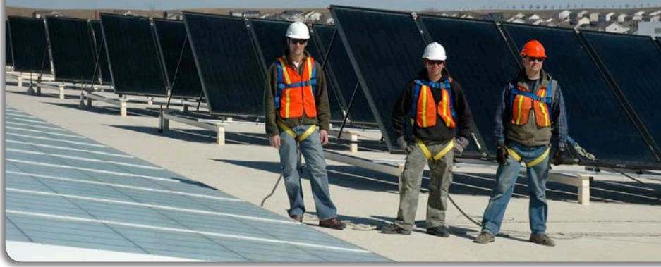
Atop the Adams 12 Schools' Veteran's Memorial Aquatic Center in Thornton, 102 collectors provide up to 60 % of pre-heating for an Olympic pool. Photo: Mike Wilson.
