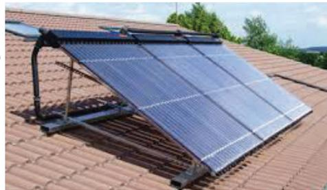
*Fig. 4.7: Roof mounting structure for flat roofs and an example of a rack mounting on tile roof to adjust pitch*
