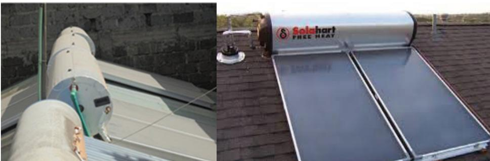
Figure 6.4: Storage tanks and collectors mounted on rooftops
