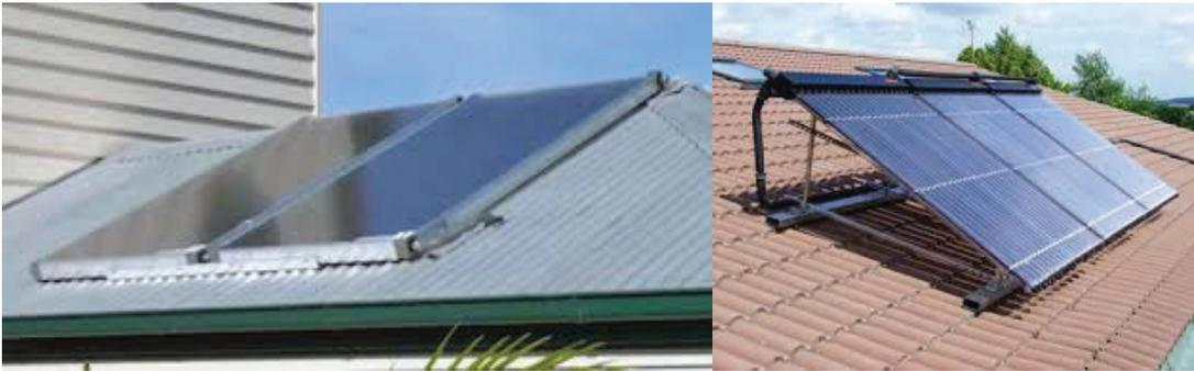
Figure 6.3: Collector and evacuated tube mounted on roof tops
