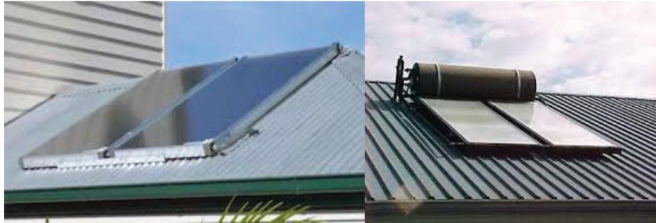
Figure 6.2: Flat Plate collector mounted on ordinary galvanized and box-type iron sheet roofs (Refer to Figure 5.9 for installation guideline)
