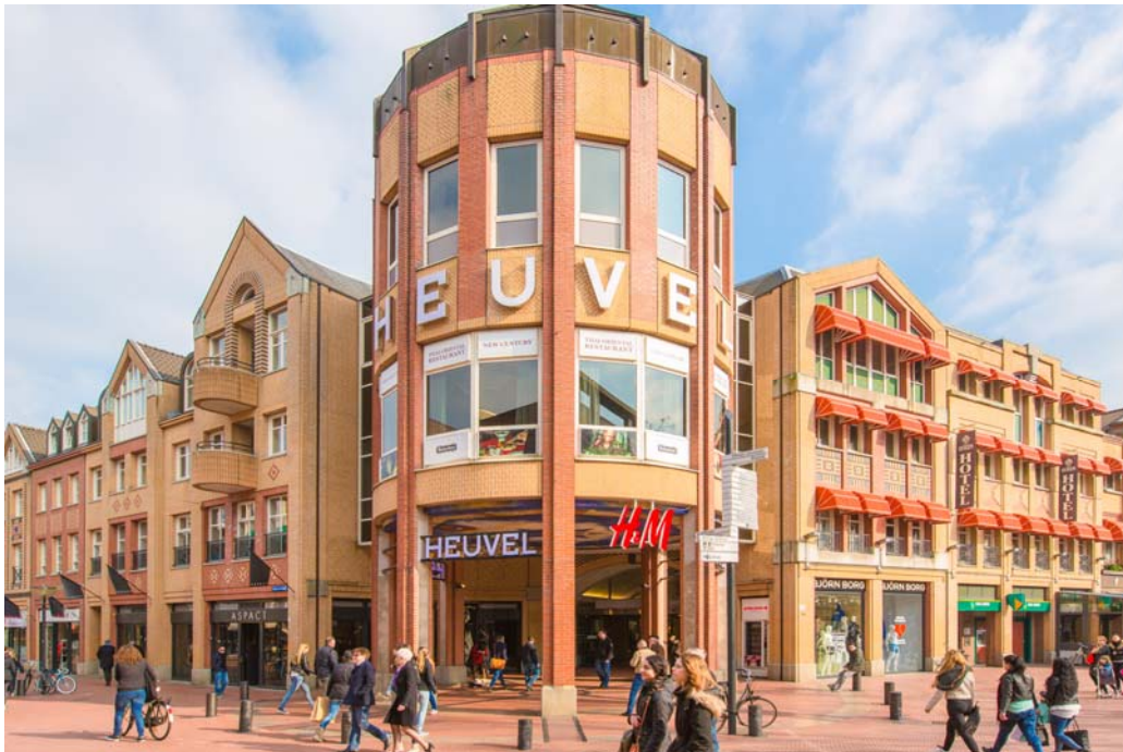
Figure 1 Shopping mall Heuvelgalerie Eindhoven (in 2015 the name Heuvelgalerie was changed in Heuvel)
