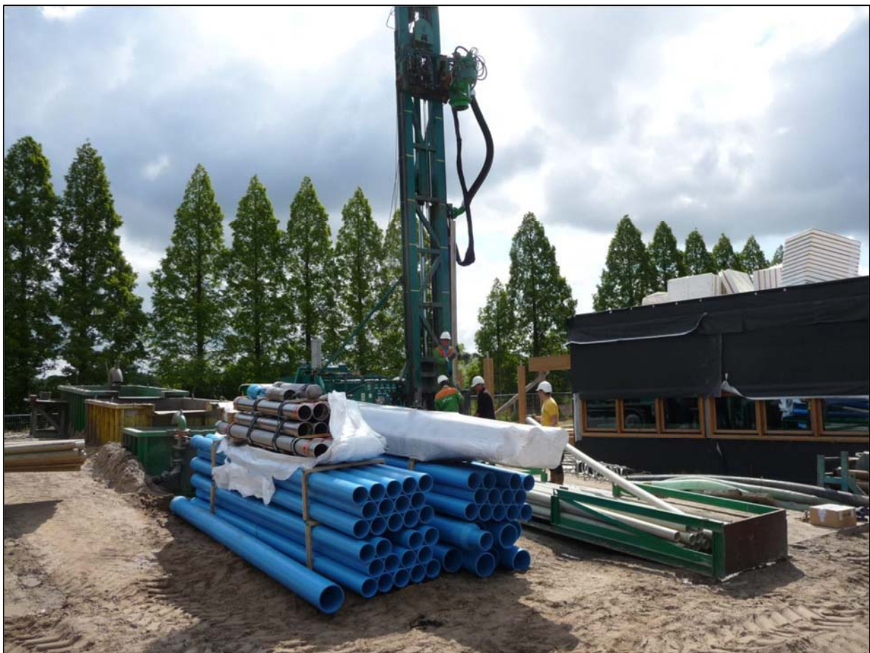
Figure 2.5 Picture from drilling site at the NIOO HEATSTORE case study in the Netherlands (IF Technology)
