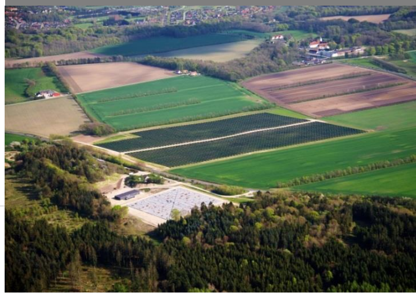
Fig. 4 Large-scale system of solar collectors with thermal energy storage cooperating with district heating in Dronninglund, Denmark. Source: PlanEnergi
