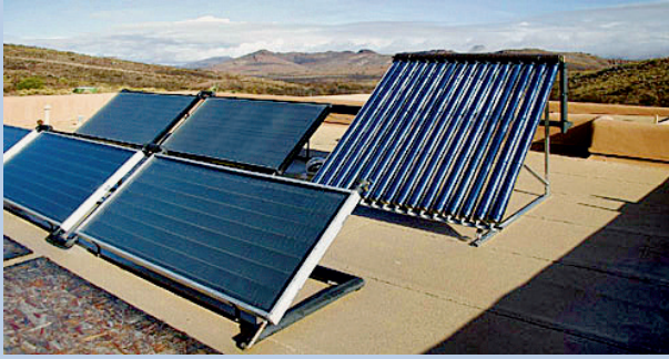
Figure 2: Flat-plate solar collectors (left) and evacuated tube collectors (right) installed on a single roof
