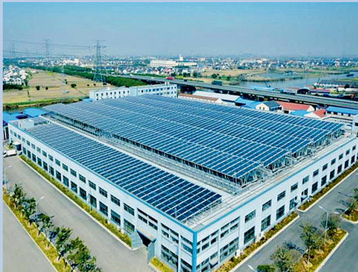
Figure 8: Installation of 7 460 m 2 of ETC in a printing and dyeing plant in China
