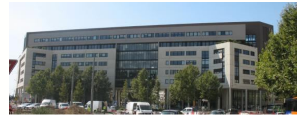
Building A view
