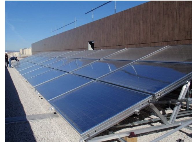
Picture of the collector field
