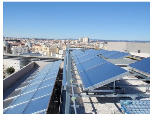
Solar collector fields in drainback mode
