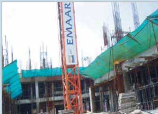
Figure 4 Safety nets at construction site
