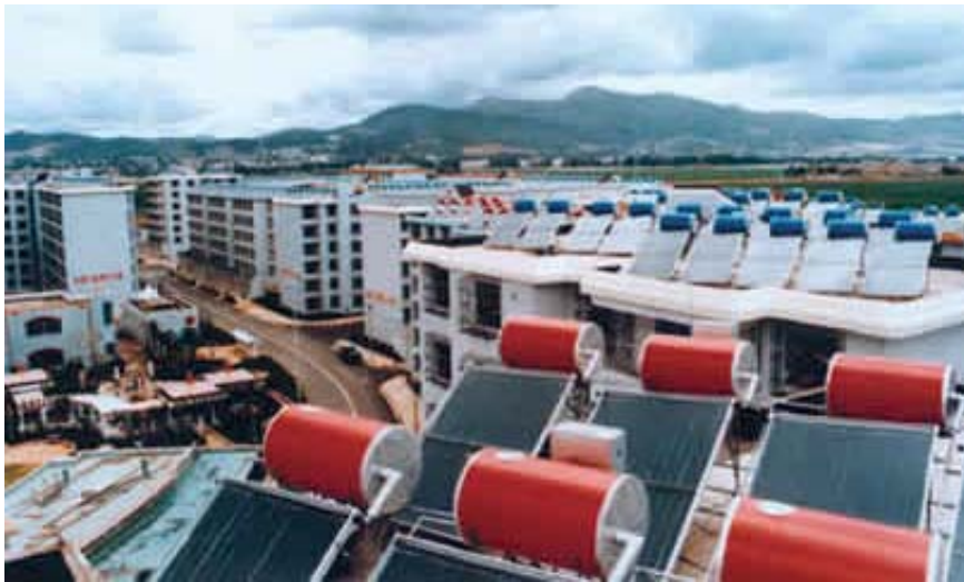
SWH systems are often installed on the roofs of residential buildings in China
