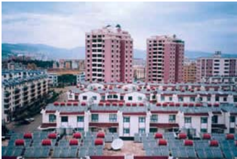
SWH systems are often installed on the roofs of residential buildings in China
