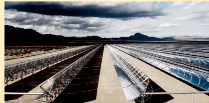
Line Focus: The Ausra Line Focus demonstration in Australia.
