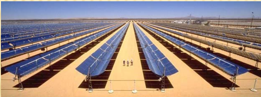
Parabolic trough collectors and foundations for the molten salt tanks of ANDASOL 1.
