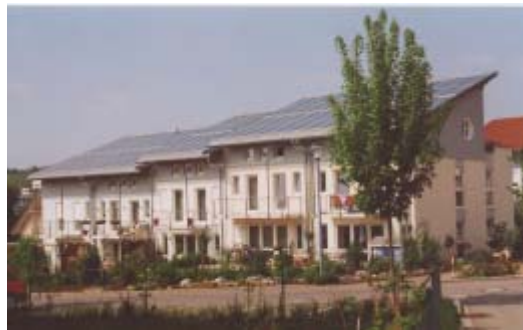
Large, roof-integrated flat plate collector split system in Germany
