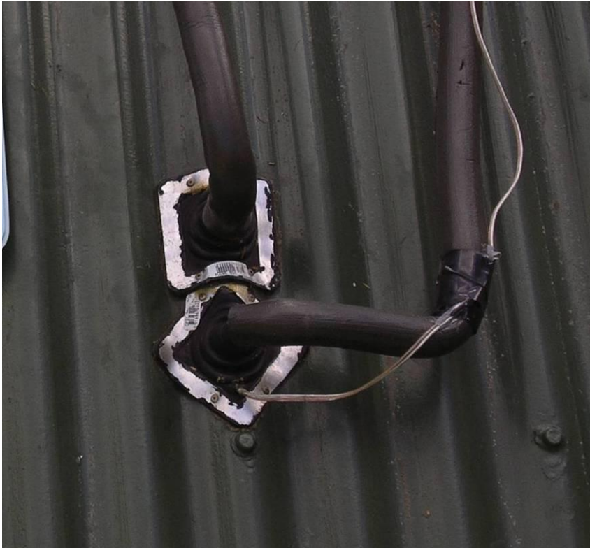
Figure 5. The lagging has been painted to match the roof – no UV damage.
