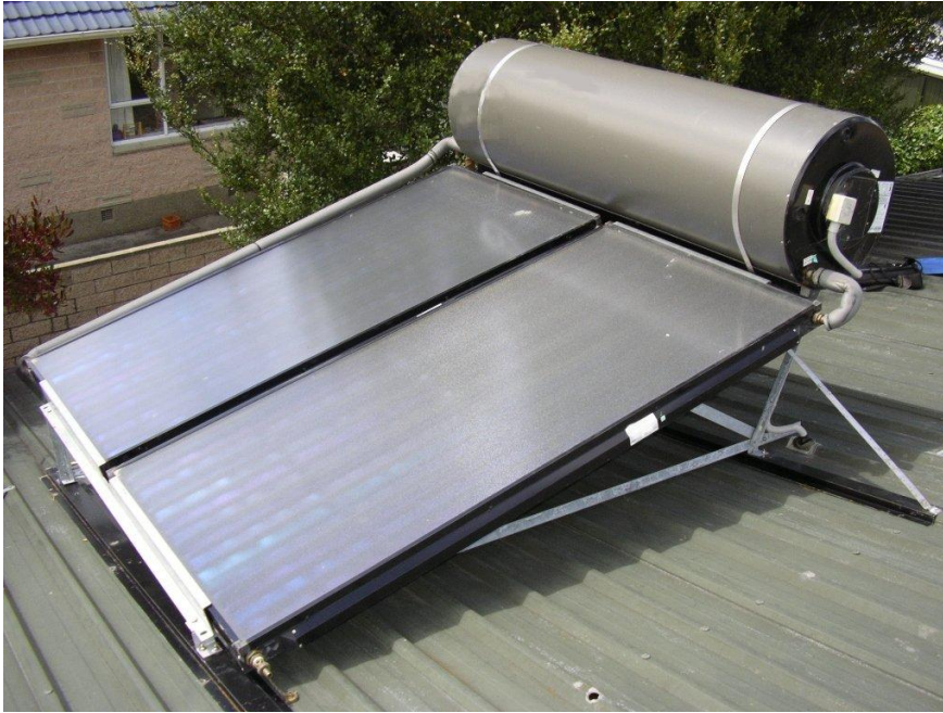
Figure 49. A large sheltered area exists under this collector.
