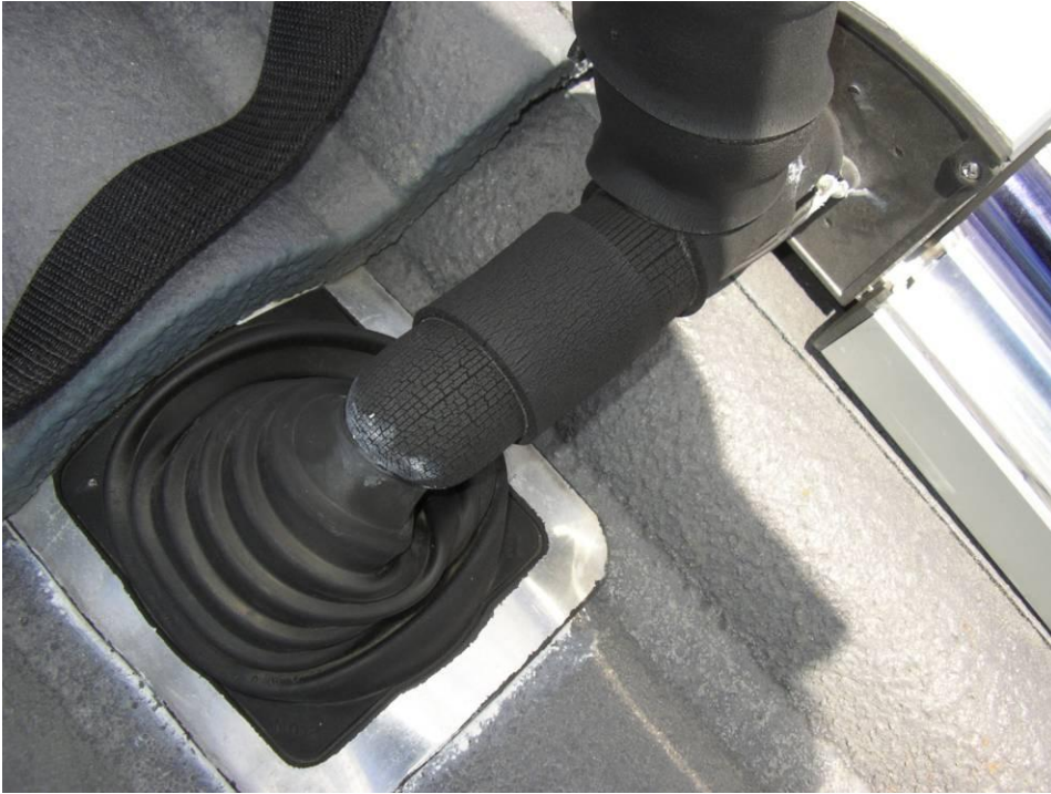
Figure 9. This is a very tidy job, but needs UV protection.
