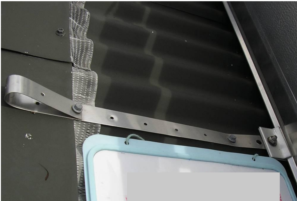
Figure 18. It is not clear whether the left fastener is tight.
