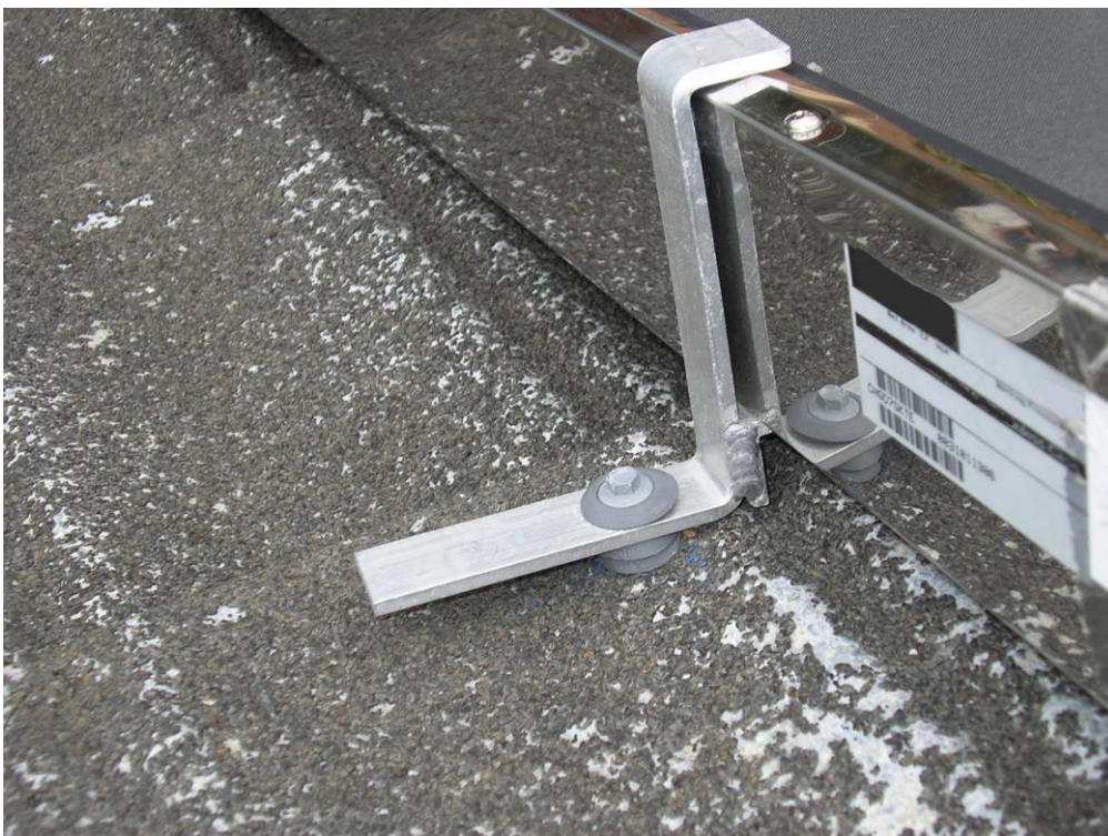
Figure 20. It is uncertain whether this bracket is tight on the stack of isolating washers.
