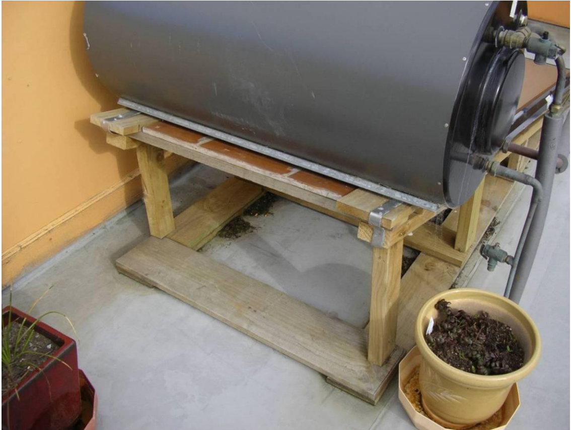
Figure 15. This tank frame is not mechanically held down at all.
