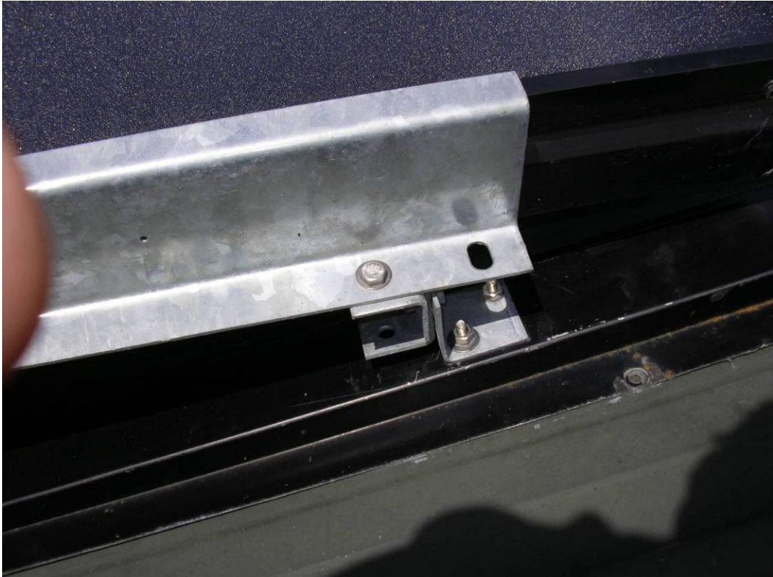
Figure 32. Stainless steel bolts, galvanised steel roof and brackets, no separators.
