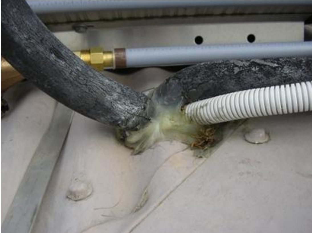
Figure 43. Degradation of lagging, unprofessional penetration sealing.
