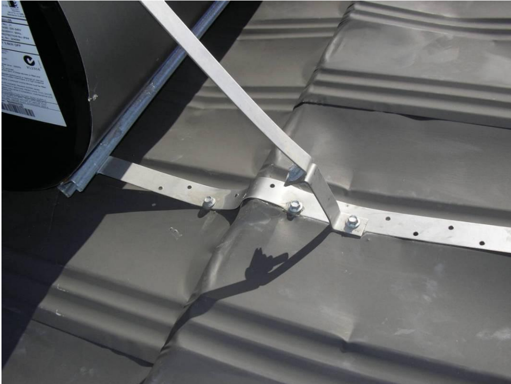
Figure 24. Stainless steel straps, sharp edges, galvanised screws, in contact with damaged roof.
