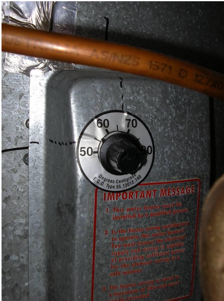
Figure 53. Thermostat set at 56°C as owner’s manual recommends.
