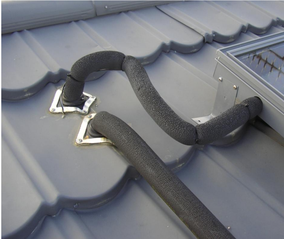
Figure 7. Note the checking of the surface of the lagging.
