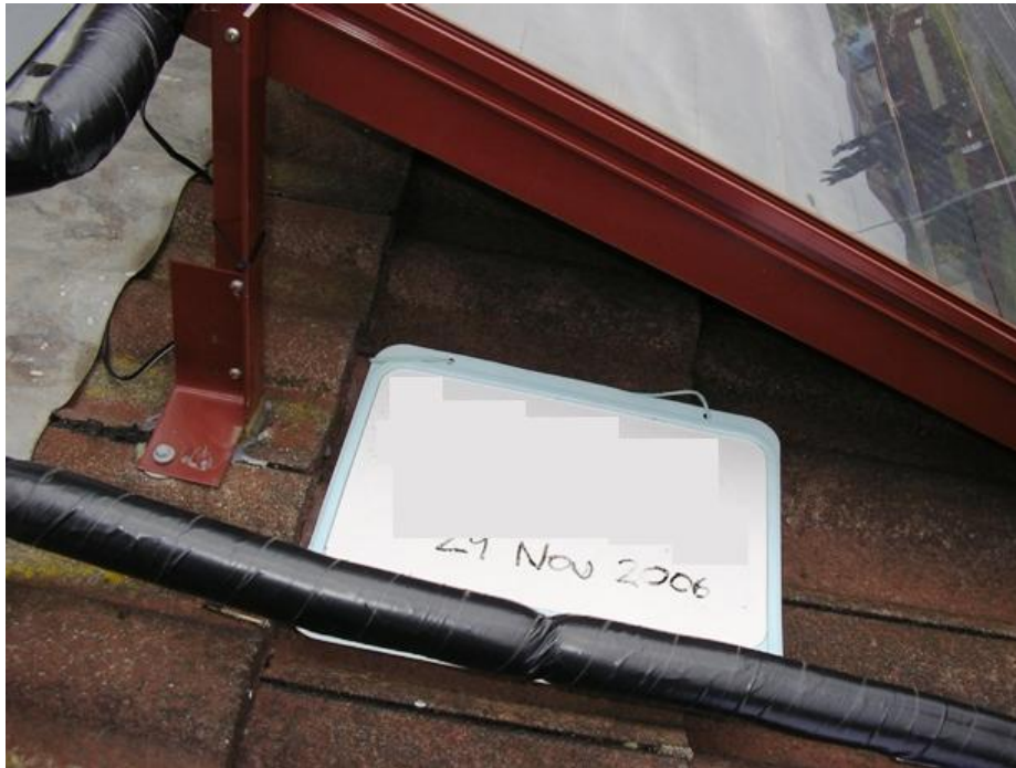
Figure 2. Unwashed area under collector can accelerate corrosion of roofing.
