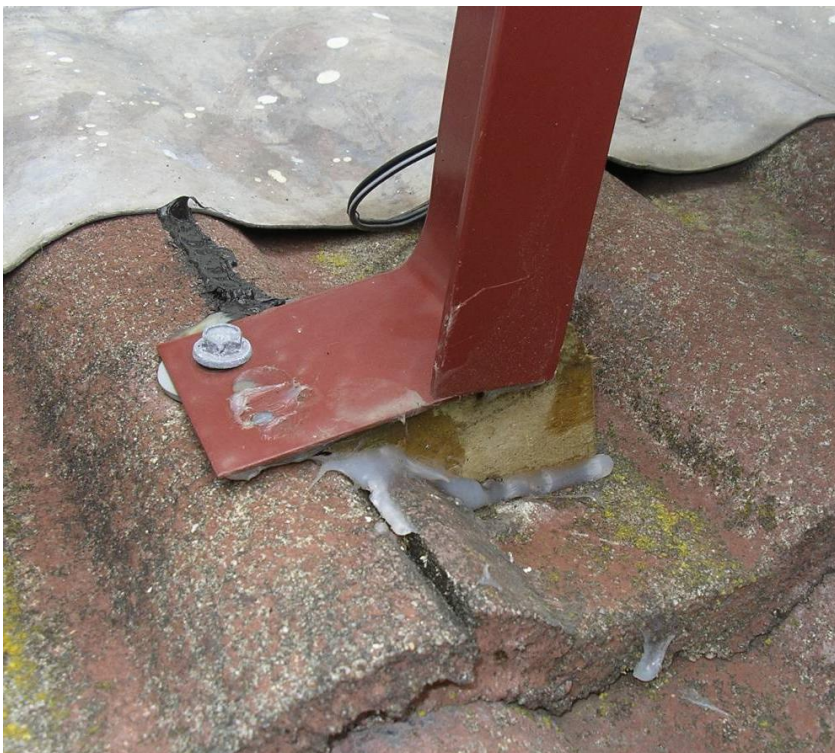
Figure 22. Fibrous board will swell further and bend bracket/break tiles.
