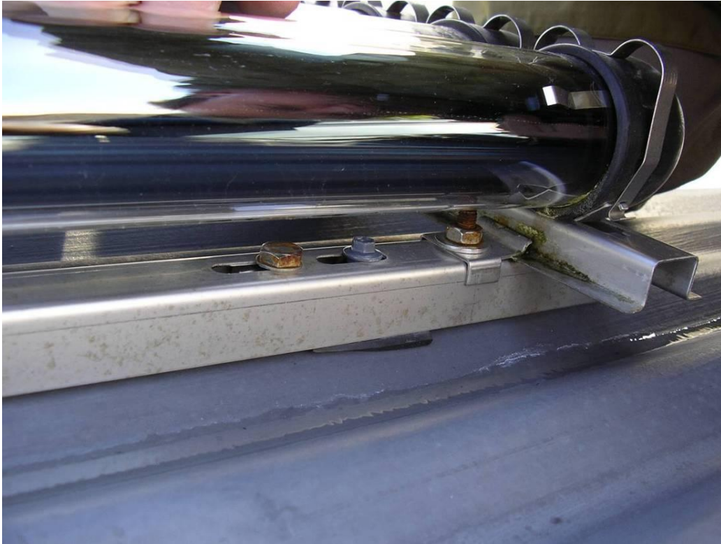
Figure 26. Separator under stainless steel channel – rust on stainless steel bolts is manufacturing fault.
