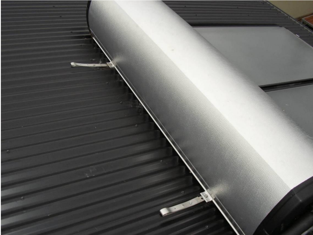
Figure 34. Stainless steel straps with zinc-coated screws used unseparated from a coated zinc-aluminium alloy roof – if the paint coating is broken, corrosion of the roofing will occur.
