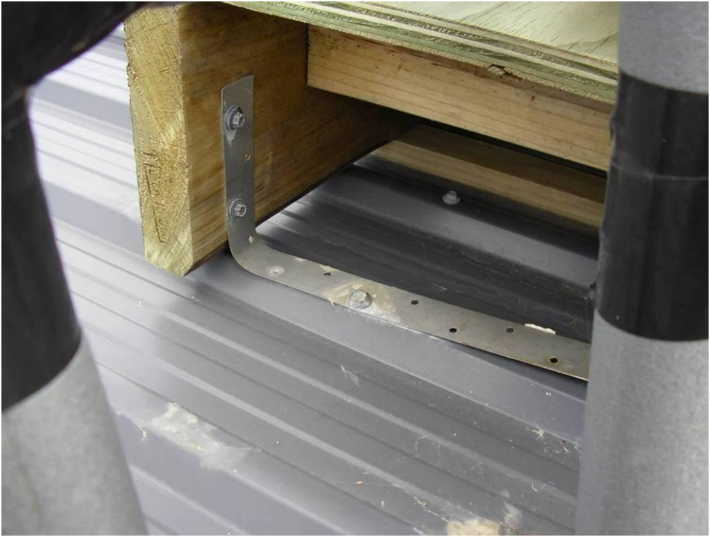
Figure 31. Stainless steel strap, galvanised screws, treated timber (holds moisture).
