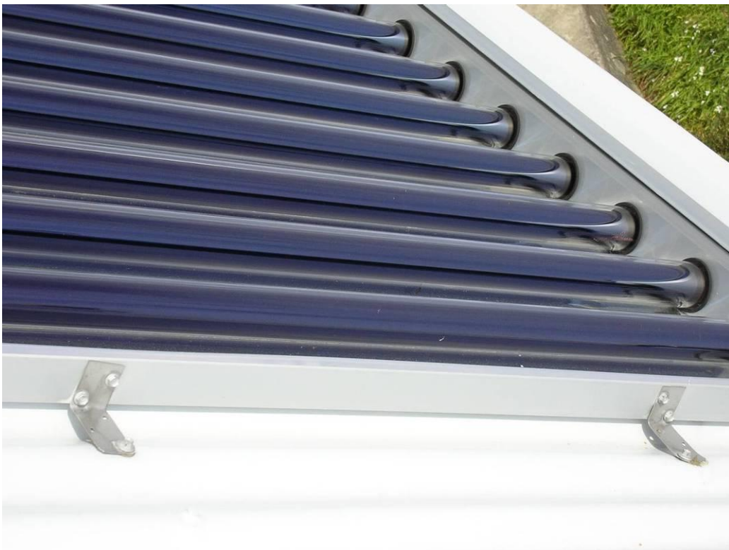
Figure 27. Stainless steel brackets with galvanised screws and separators.
