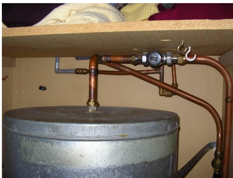
Figure 50. The tempering valve is fed from two hot supplies – the HWC and the SWH.
