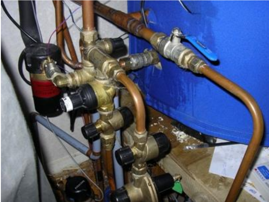
Figure 4. Complicated valve arrangement – the cylinder is within the blue cover to the right.
