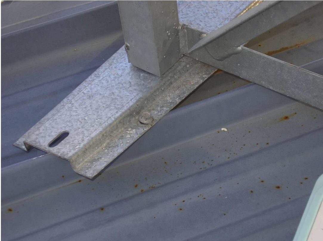
Figure 11. Note rusty swarf. See also Figures 19 & 42
