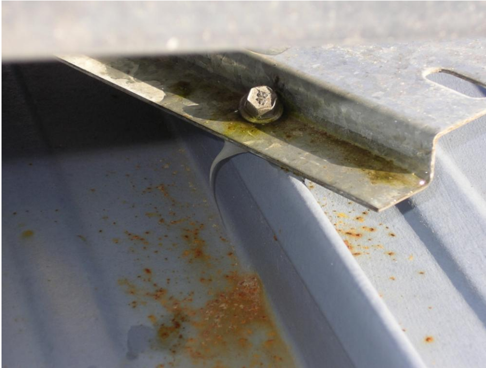
Figure 19. Four screws hold this tank/frame/collector onto the roof – each like this.
