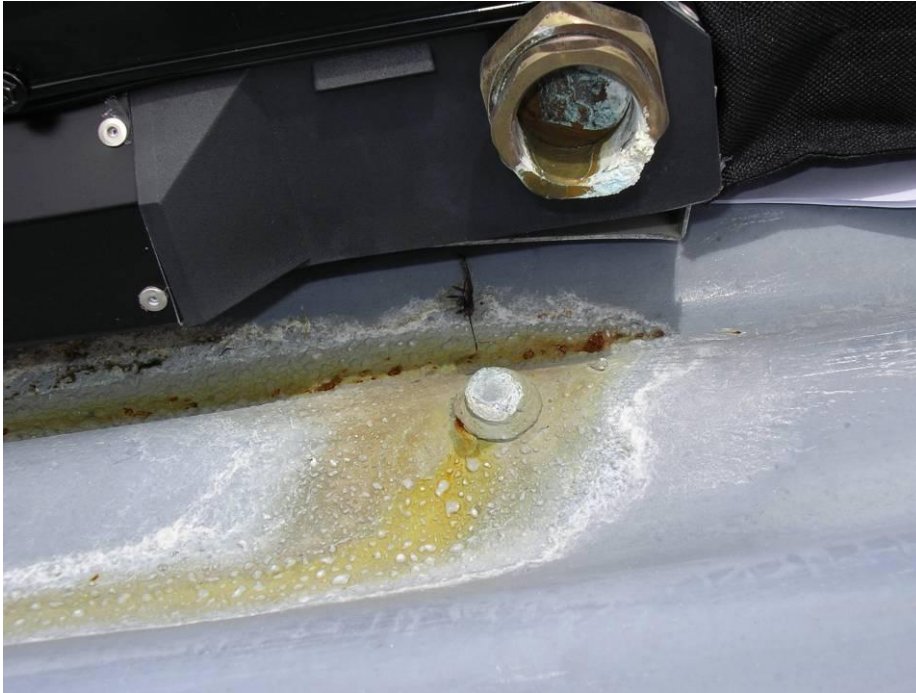
Figure 14. Leaky washer has caused corrosion of roof.
