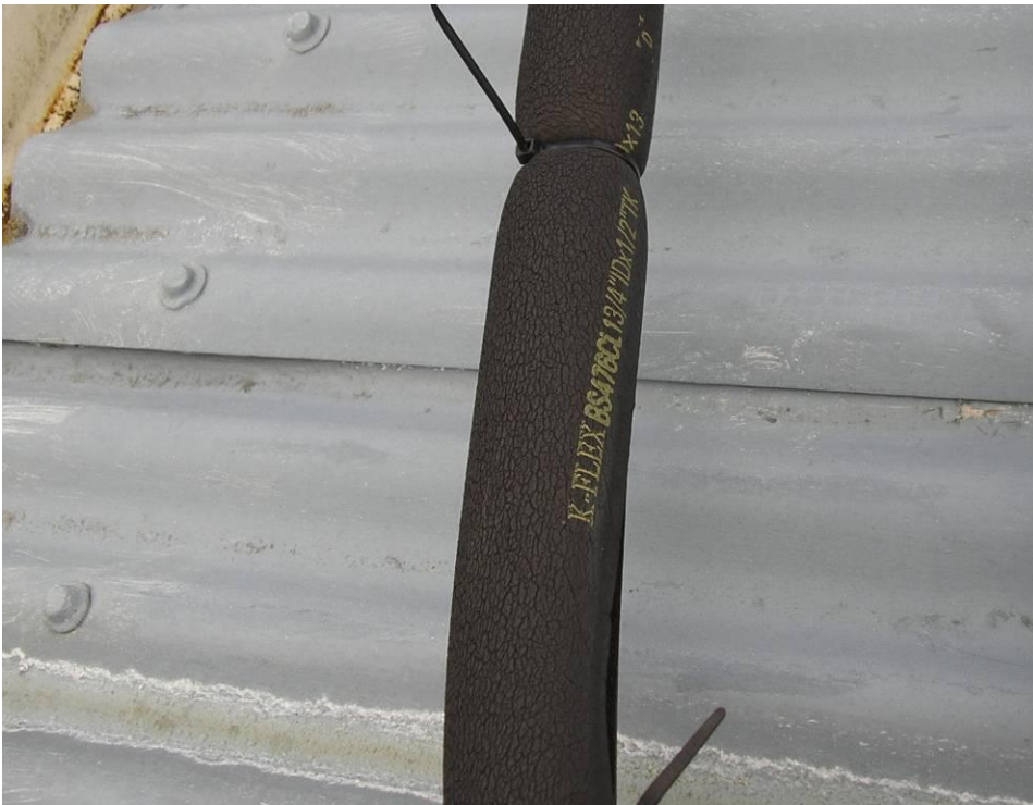
Figure 10. Surface checking,
