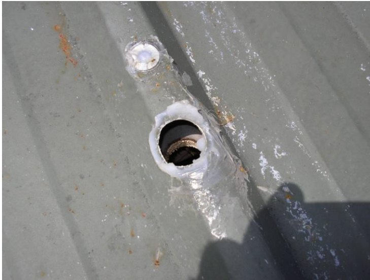
Figure 51. Hole left after reorienting collector by 90° – it is 25 mm in diameter.
