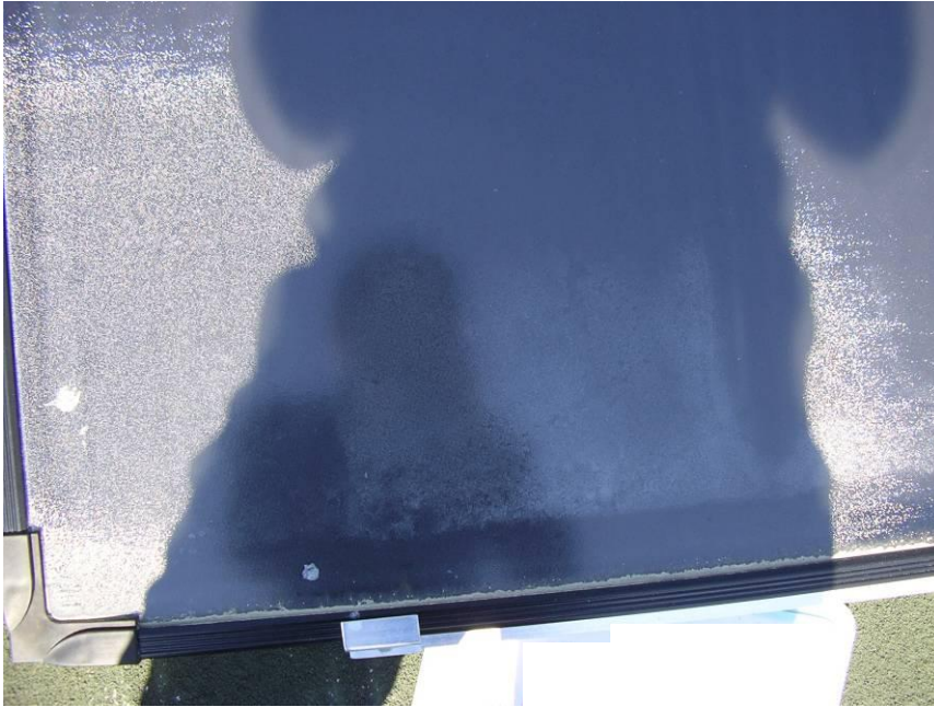
Figure 47. Condensation inside glass.
