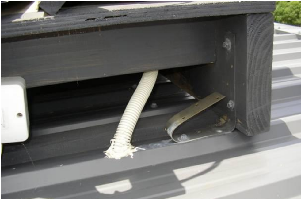
Figure 44. Dissimilar metals in contact, unprofessional penetration sealing.
