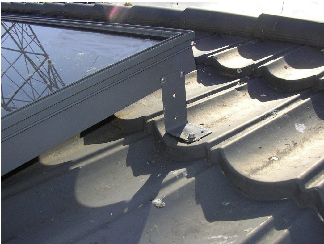
Figure 29. Painted steel bracket, with sharp edges touching roof despite separator.
