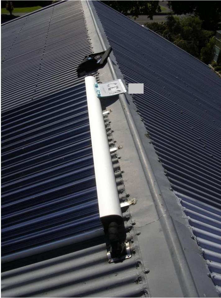
Figure 52. Collector at 120°C – note the lack of relief valve.
