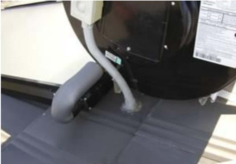
Figure 41. Good use of an electrical isolation switch glued to the exterior of a roof-top cylinder. Note, however, the poor flashing for the conduit passing through the roof.
