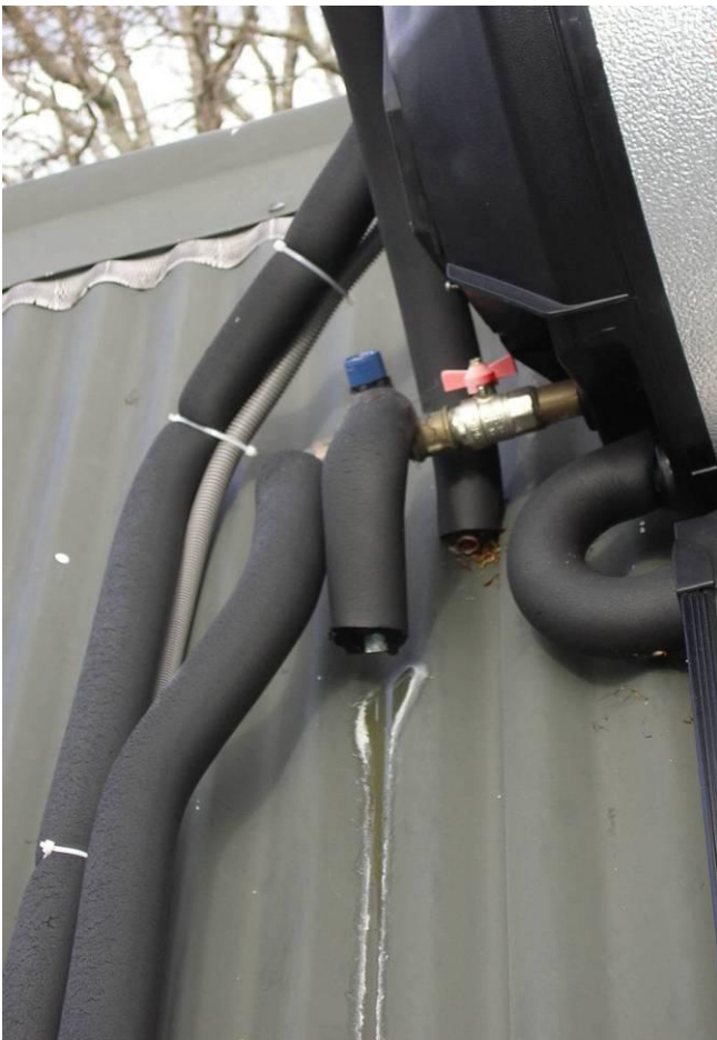
Figure 13. Cold water expansion valve in copper pipe has caused corrosion lower on roof.
