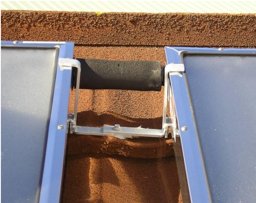
Figure 17. Good to see connect pipe lagged – but needs UV protection
