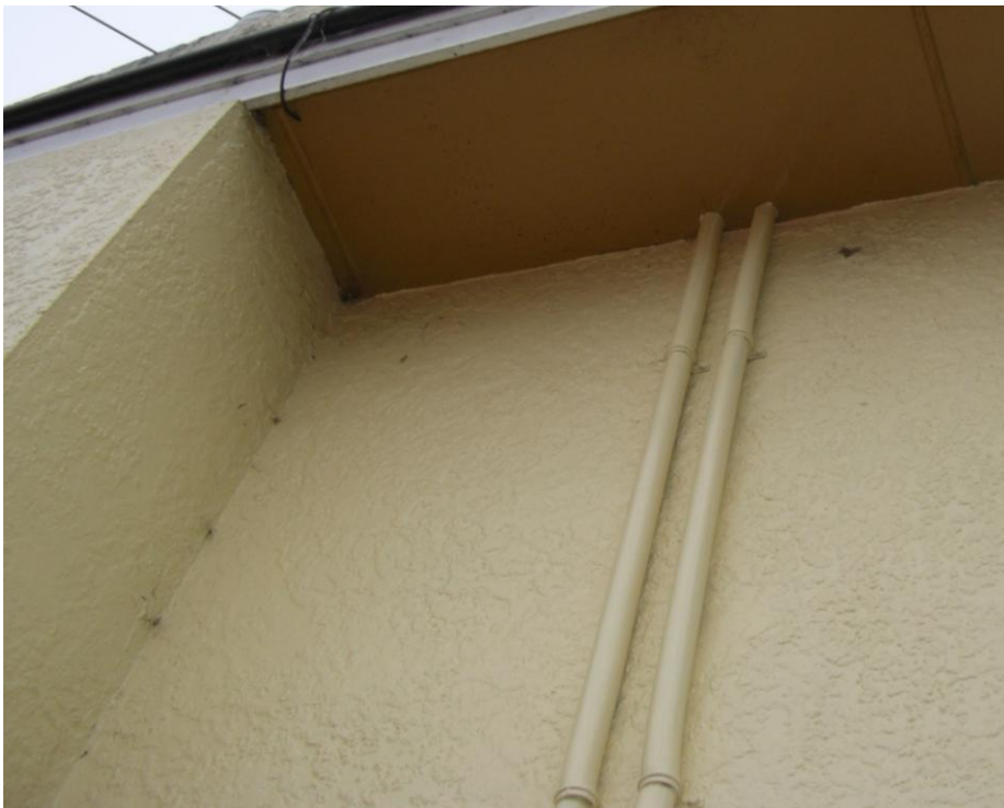
Figure 8. This lagging (north wall) has been painted – no UV damage.
