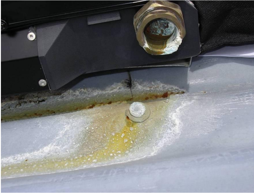
Figure 45. A leak has directed copper containing water onto the roof, corroding it.
