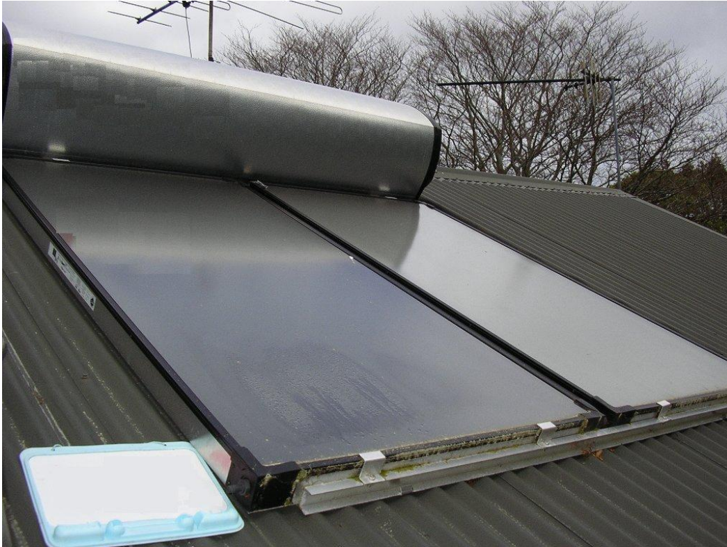
Figure 3. Water trapped inside collector.
