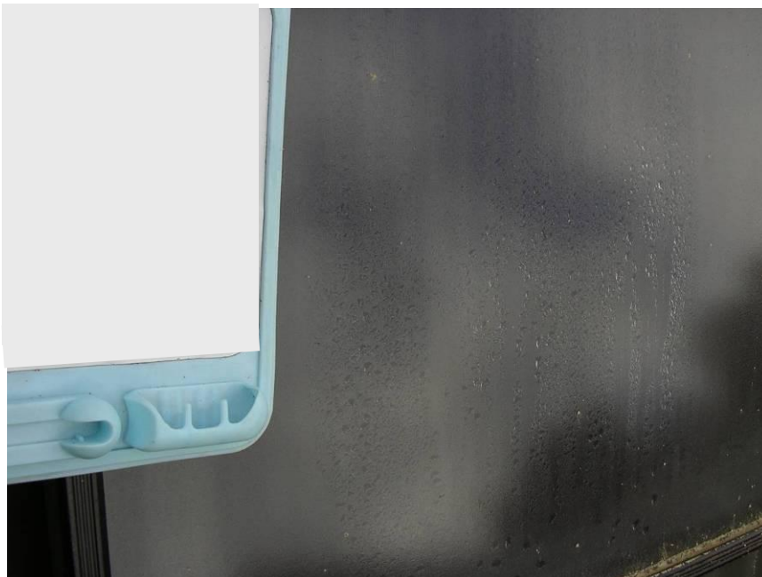
Figure 48. Condensation in collector.
