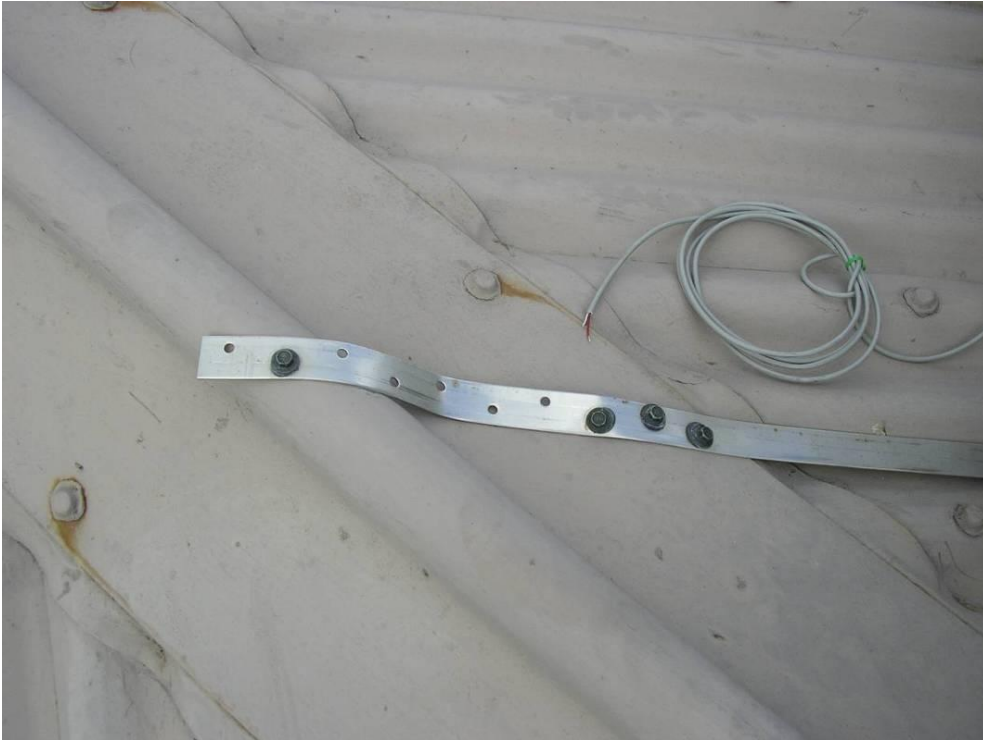
Figure 30. Painted galvanised screws, stainless steel strap, painted roofing, no separators.
