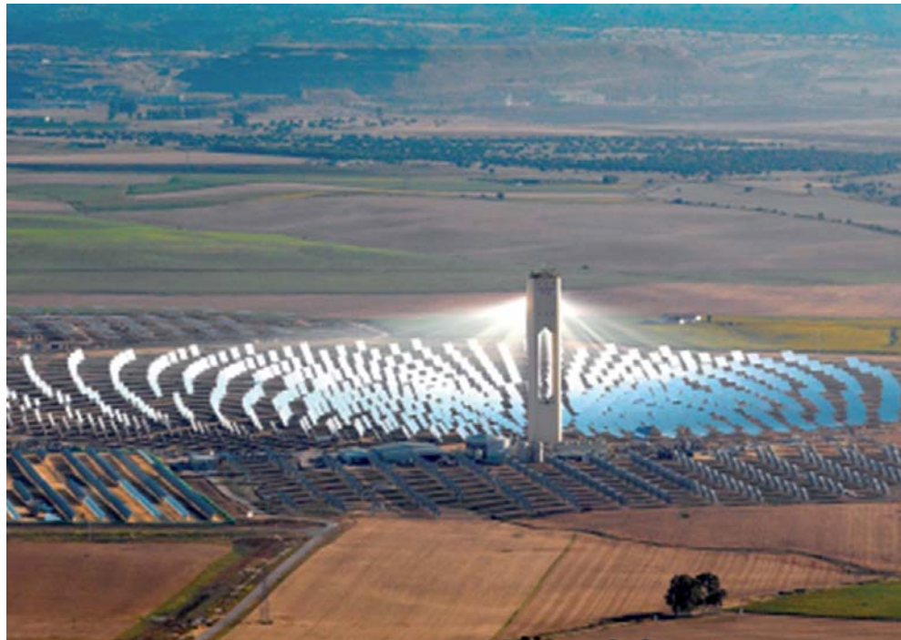
Figure 1. Power plant PS10 in Sevilla. Owned by Abengoa.
