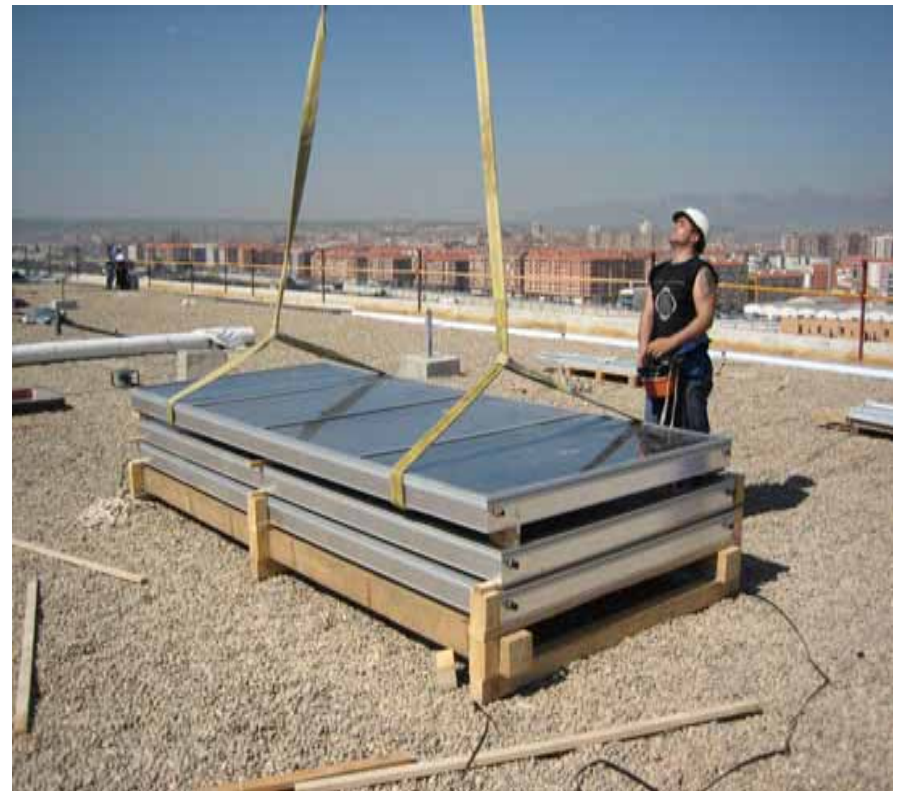
Example of large flat plate collectors
